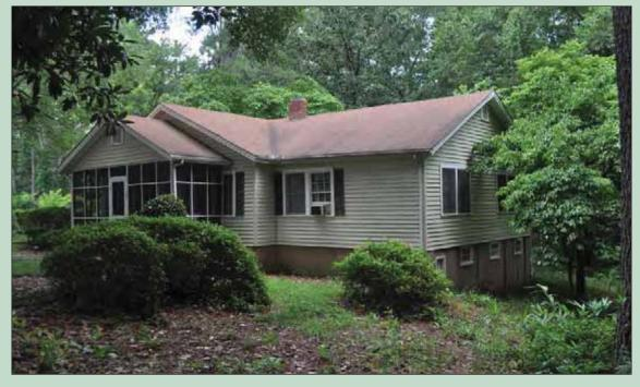
Asphalt shingles top the roofs of the main massing, additions, and porches. A single brick chimney is visible in the ridgeline of the side ell. No additional chimneys were identified during the field survey.
