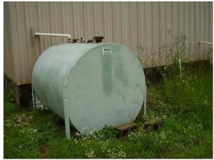
**Photo #12** View of an used oil AST behind William's Automotive.
