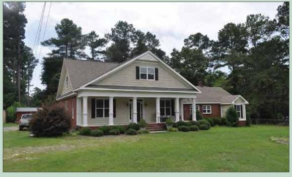
The entire roof of the original building and its large addition is covered in asphalt shingles. The ridgeline of the original building's main massing hosts two brick chimneys.
