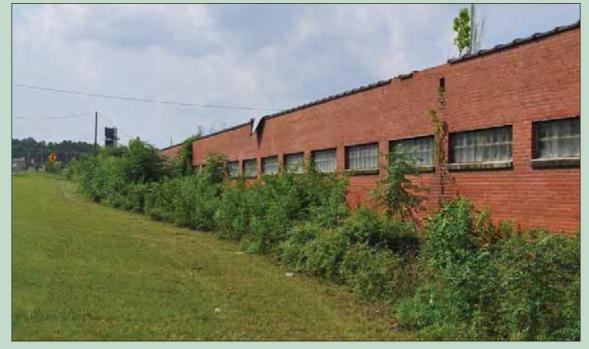
Symmetrically spaced window bays and an offset truck bay mark the rear elevation of the production building (Figure 28A). Covered by a corrugated metal door, the truck bay sits between two window bays near the east end of the rear, or south, elevation. The window bays on this elevation also sit atop poured concrete sills and feature paired, metal, multi-light awning windows. Here, windows left in an open position and missing panes expose the building to invasive elements.
