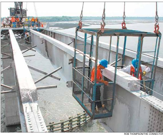
Construction workers are lowered into place to remove a damaged beam as part of the repairs to the McTeer Bridge on May 18, 2007.
