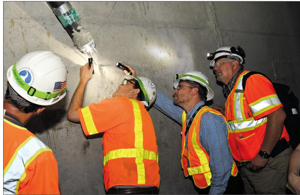
**SCDOT, Federal Highway, Florida DOT and other experts familiar with the box truss bridge design inspected the damage to determine the cause of the cable break. The team also managed the repair operations and inspected the work as it was done.**
