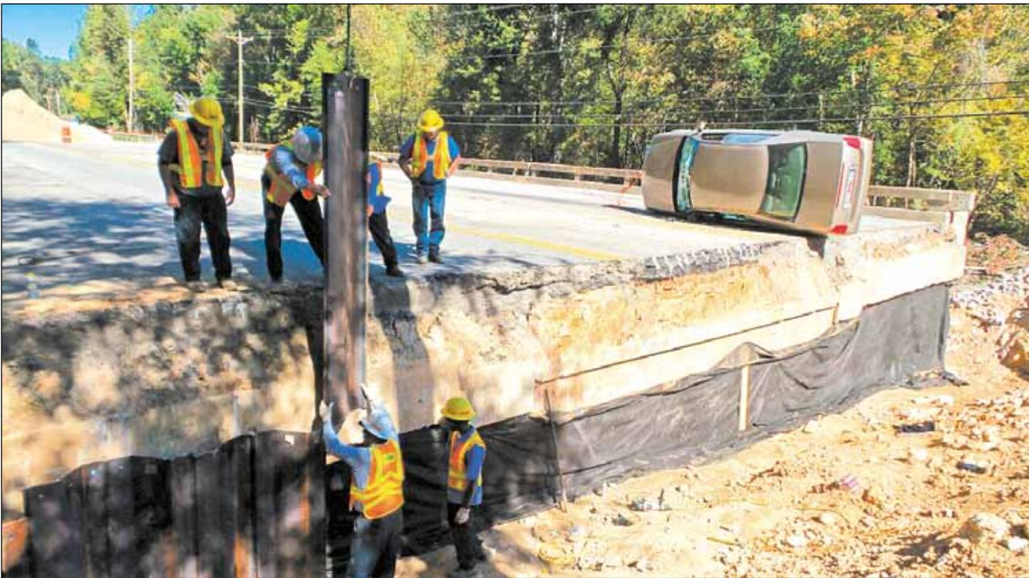
**John Taylor of Aiken Maintenance guides a sheet piling into place with the help of his team doing work on the washed-out bridge headwall on Fairfield Road in Richland County. The work is part of SCDOT's ongoing flooding repairs across the state.**
