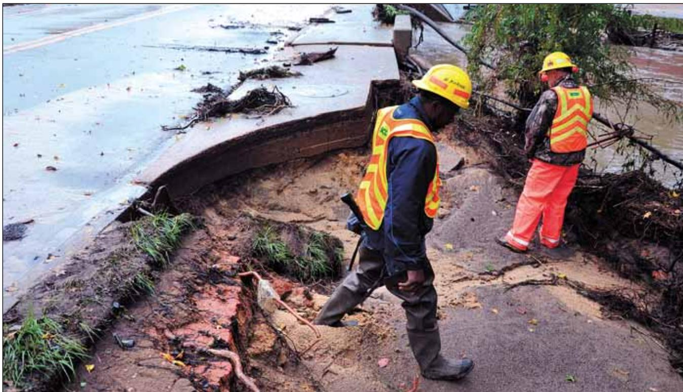
**The District 1 Bridge inspection crew examines and monitors the washout of sidewalk around a bridge on U.S. 1 in Lexington on Oct. 5. SCDOT crews monitored bridges statewide during the flooding.**
