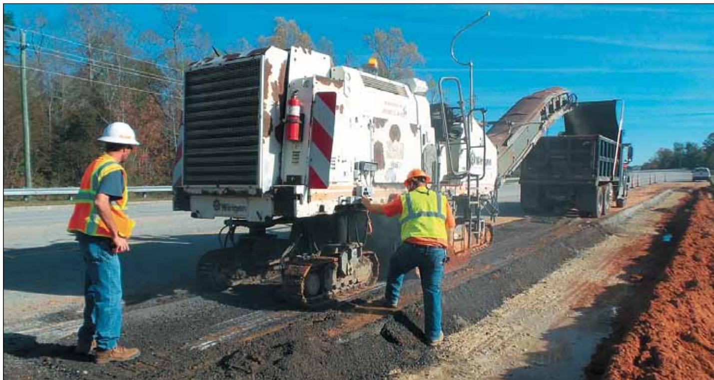
**Allen Oxendine of SCDOT's Aiken Construction unit supervises the milling operation on U.S. 521 in Clarendon County on Nov. 20. The road was being prepared for paving to complete the repairs of a washed-out section of the road damaged by the October flooding.**
