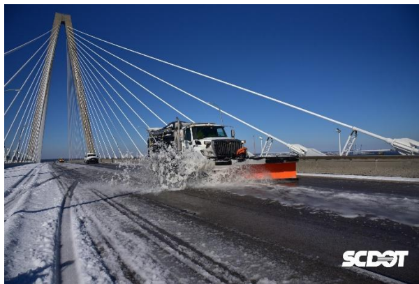
Image 5 SCDOT clears the Ravenel Bridge in Charleston
