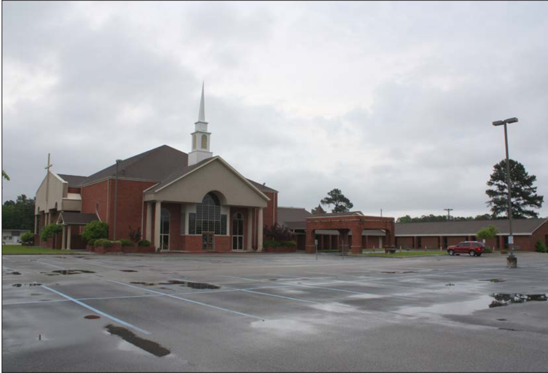
A. 1999 Sanctuary Addition and 1985 Addition, Southwest Oblique
