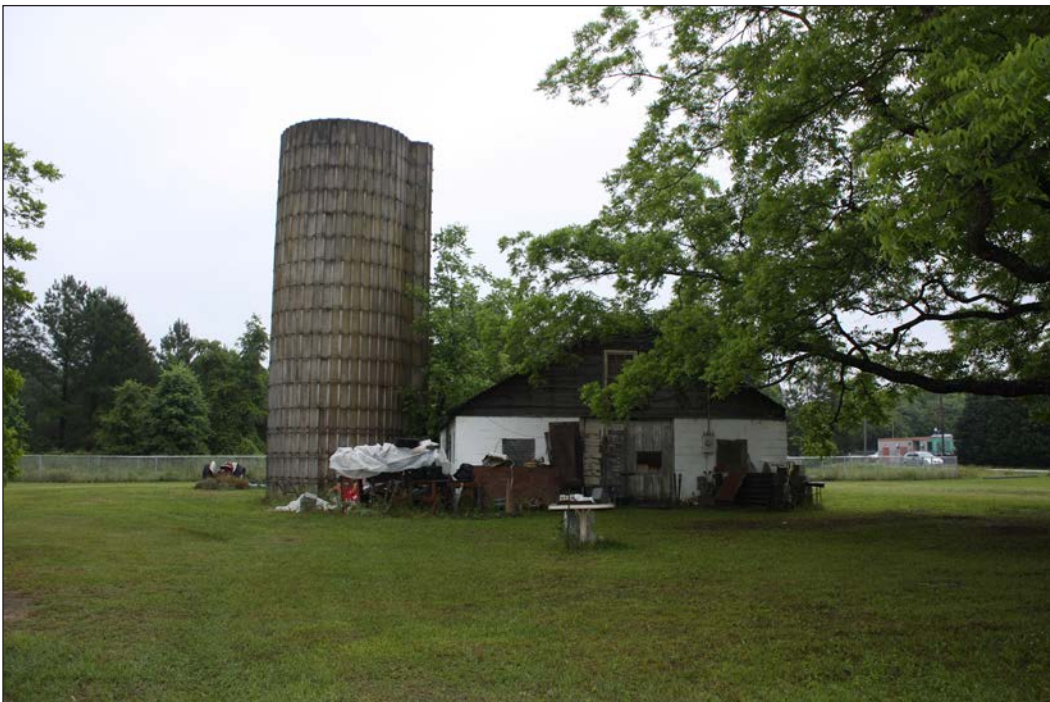
B. Barn and Silo, Looking East
