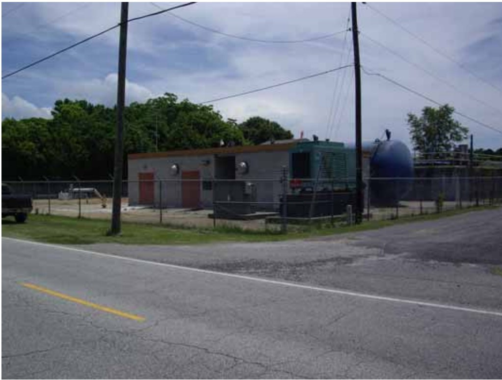
Photograph 11 – View of City of Florence Water Treatment Plant.
