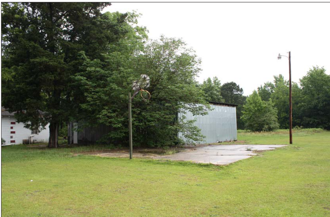
B. Outbuilding, Southeast Oblique
