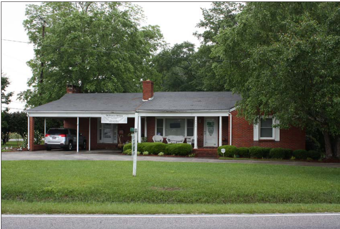
B. Facade, East Elevation
