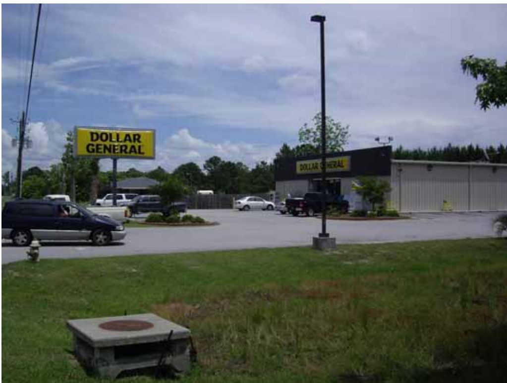
Photograph 14– View of Dollar General site.
