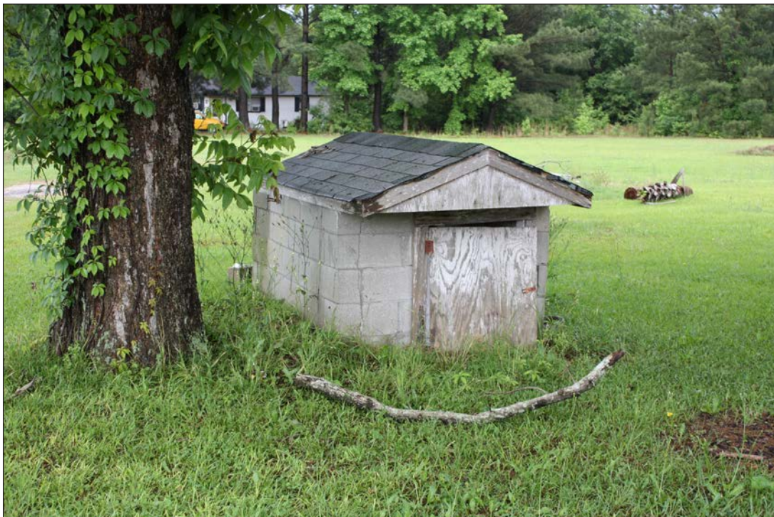
B. Well House, Northeast Oblique
