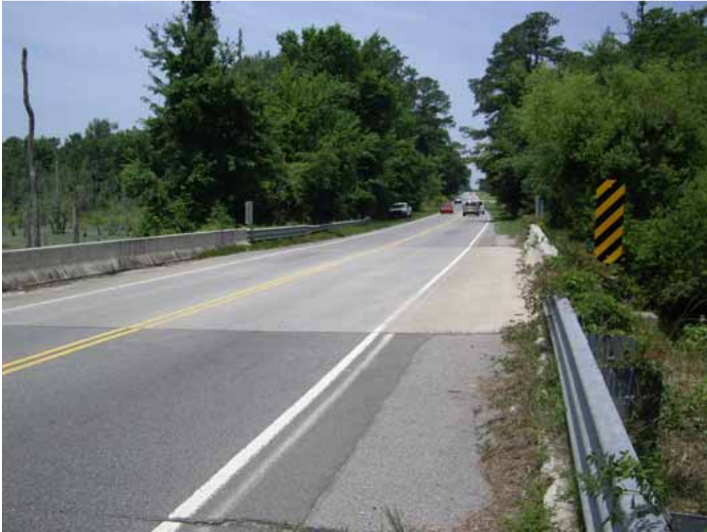
Photograph 1 – Top view of the Alligator Road (S-21-107) Bridge over Alligator Swamp.
