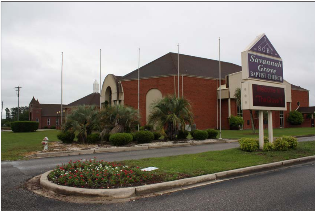
B. Roots of Savannah and 1999 Sanctuary Addition, Northwest Oblique
