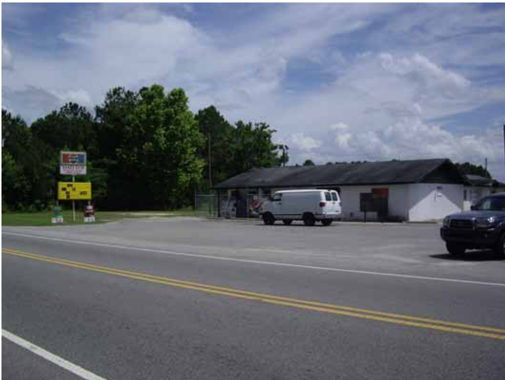
Photograph 2 – View of Dad-D-O Grocery (former Gause's Grocery).
