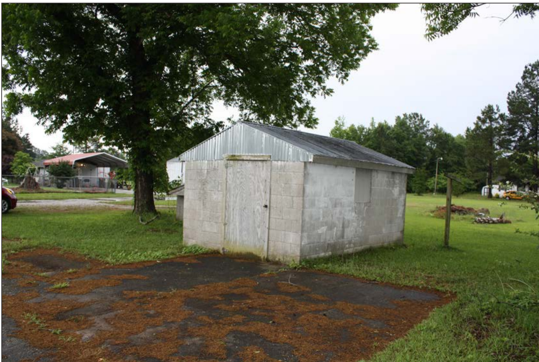
B. Shed, Northwest Oblique
