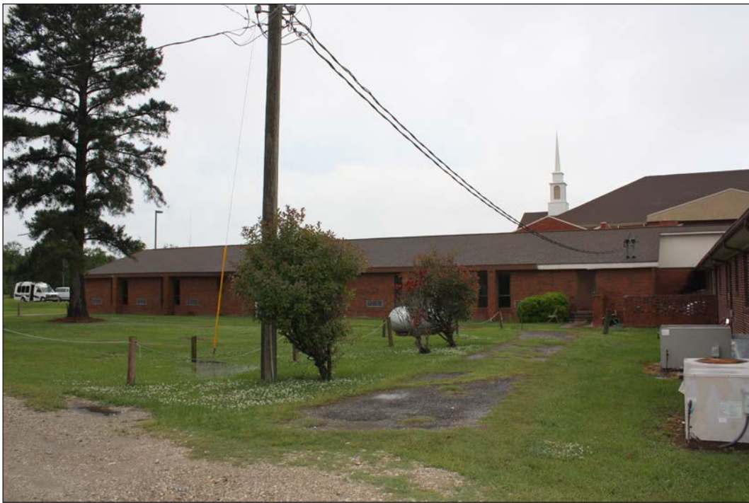
B. 1985 Addition, East Elevation
