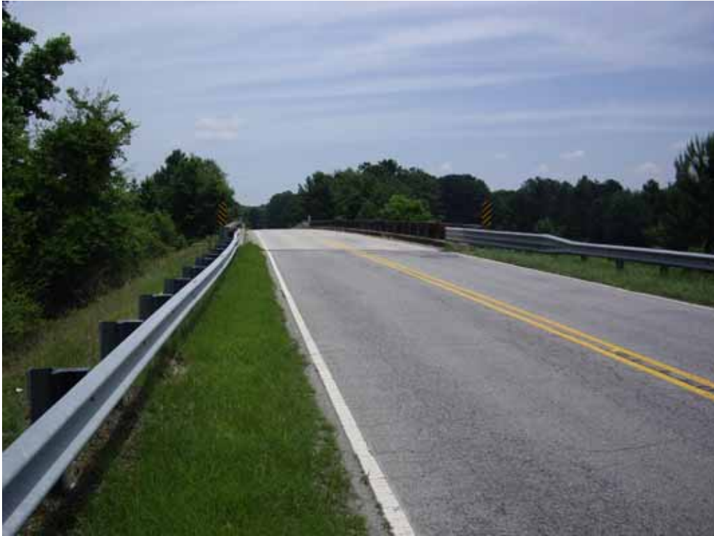
Photograph 1 – Top view of the Alligator Road (S-21-107) Bridge over I-95.
