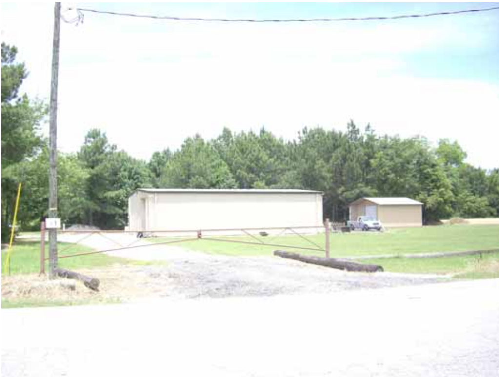
Photograph 10– View of small private garage located along the Project Corridor.
