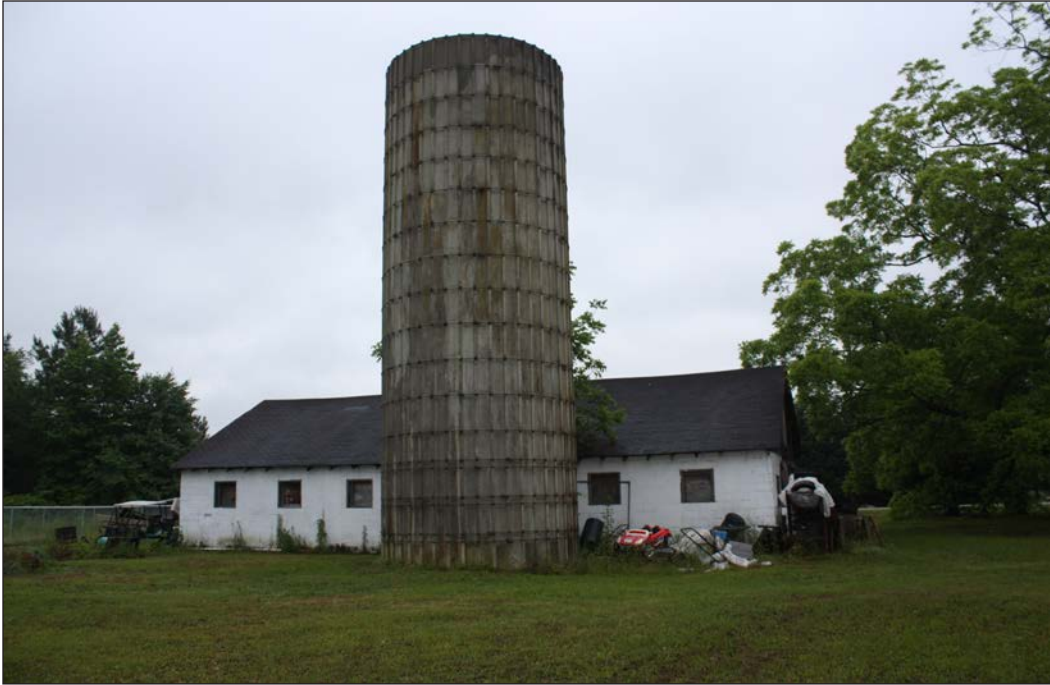
A. Barn and Silo, Looking South
