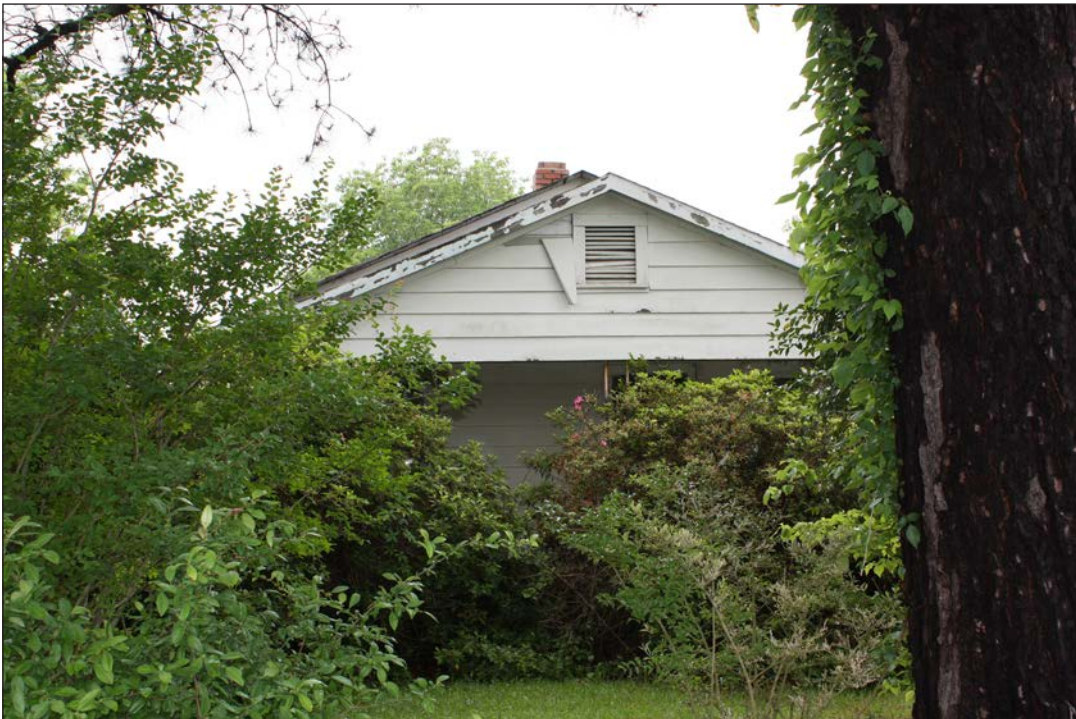
B. Facade, South Elevation
