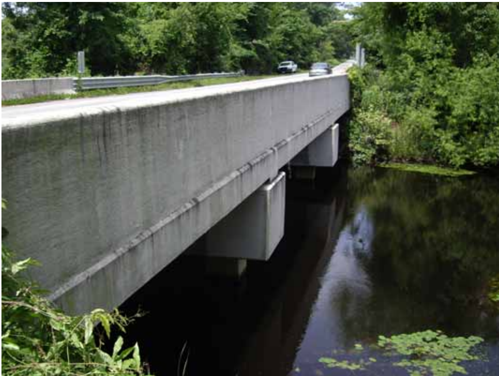
Photograph 2 – Side view of the Alligator Road (S-21-107) Bridge over Alligator Swamp.
