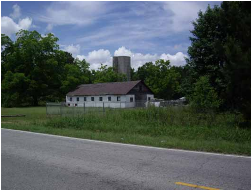
Photograph 9 – View of small private garage located along the Project Corridor.
