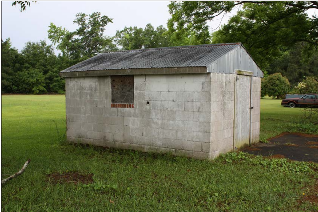
A. Shed, Northeast Oblique
