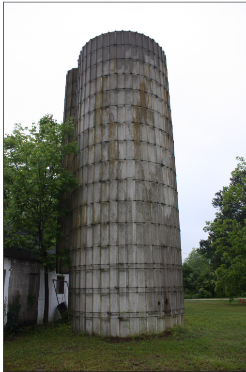
B. Silo, Looking West
