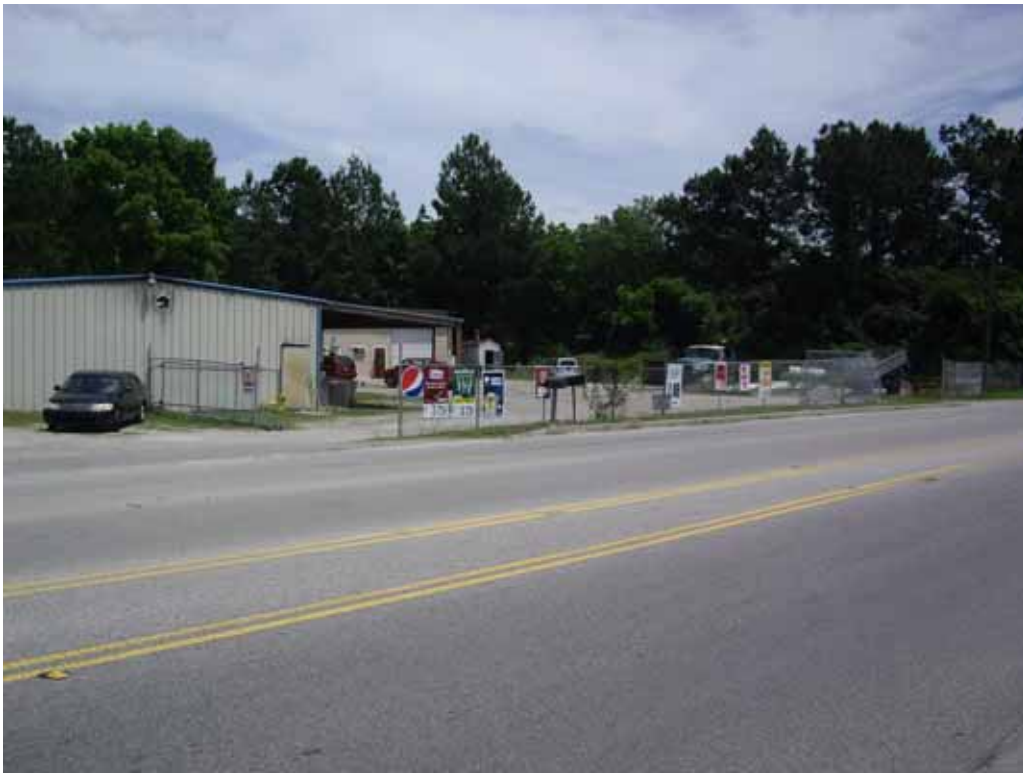
Photograph 15 – View of small garage facility located on Savannah Grove Road, near Alligator Road.
