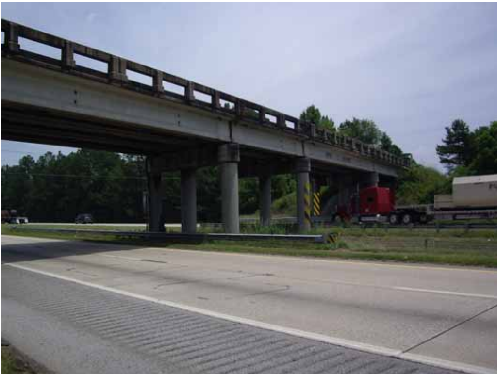
Photograph 2 – Side view of the Alligator Road (S-21-107) Bridge over I-95.
