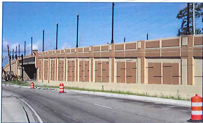
Mechanically Stabilizing Earth (MSE) walls built for the town of Mount Pleasant on Johnnie Dodds Blvd
