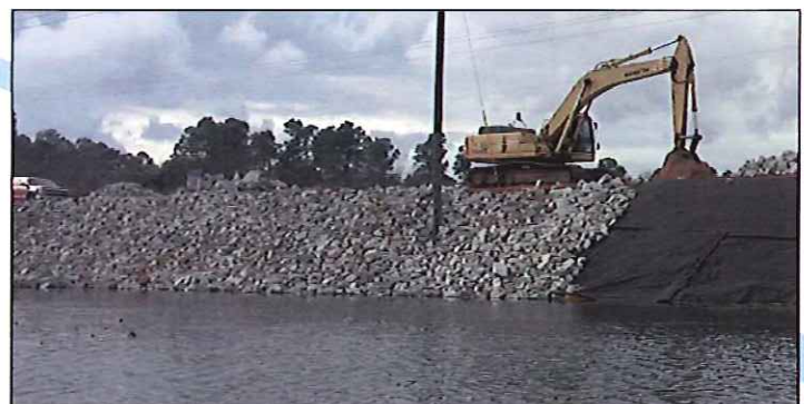
Installing rip-rap slope protection
