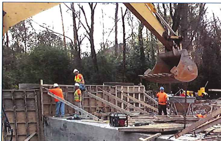
Caughman Road emergency culvert in Columbia
