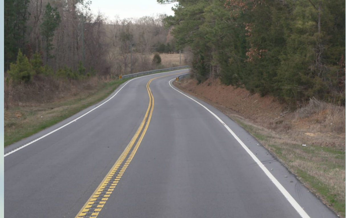
Example of Thin Asphalt Overlay
