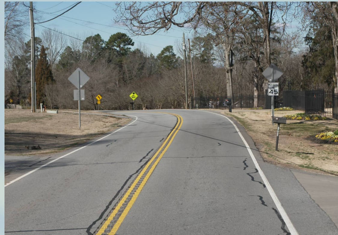
Example of Crack Seal Project
