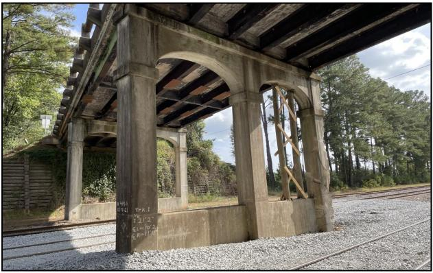
Figure 18. SHPO Site No. 5644, bridge bent detail showing recent damage and temporary repairs, looking southeast
