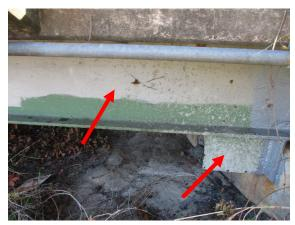
Photo 5. LBP on Gray Steel Girders and Green Steel Girder Brackets.
