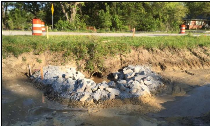
**Sediment Dam for Pipe Inlet**
