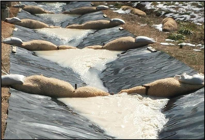
**Passive Flocculant Treatment System with Sediment Tubes**
