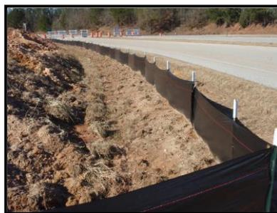
**Silt Fence with Steel Post**
