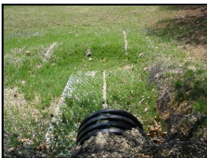
**Level Spreader for Outlet Protection**
