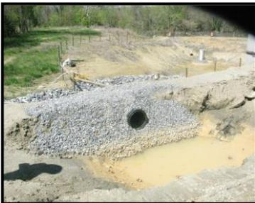
**Pipe Slope Drain Inlet with Berm**
