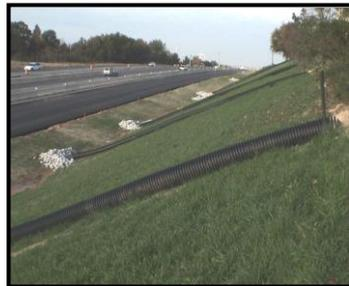
**Pipe Slope Drains**
