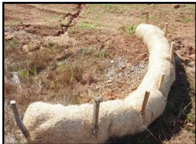
**Sediment Tube for Ditch Check**
