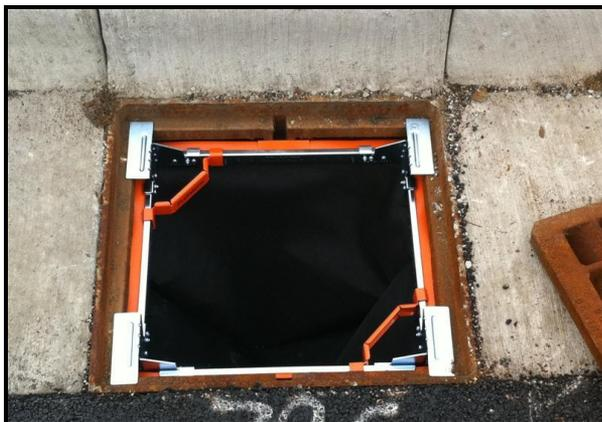
**Type G Suspended Internal Inlet Filter**
