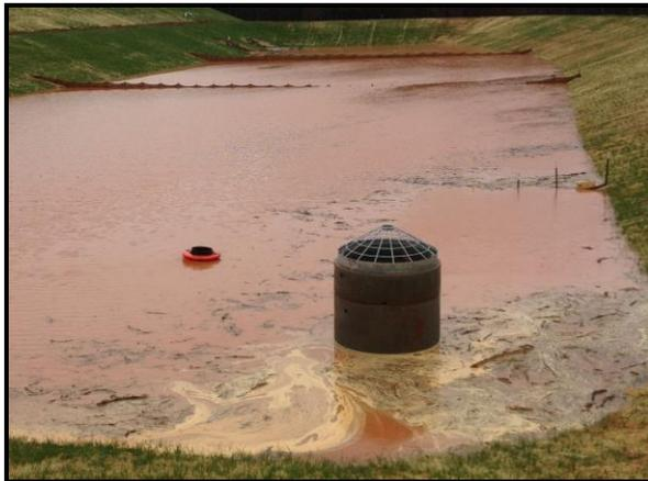
**Temporary Surface Outlet and Baffle Sediment Basin**
