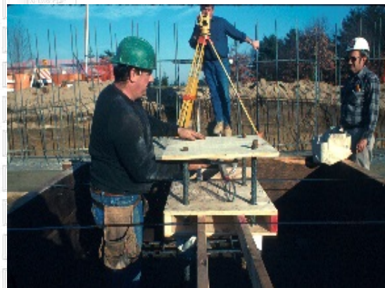
Figure 4: Templates for Columns
