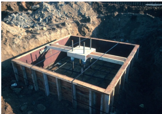
Box Jig Template for Column
