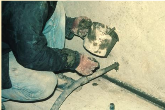
A: Pump grout into sleeve through the inlet port continuously and slowly
