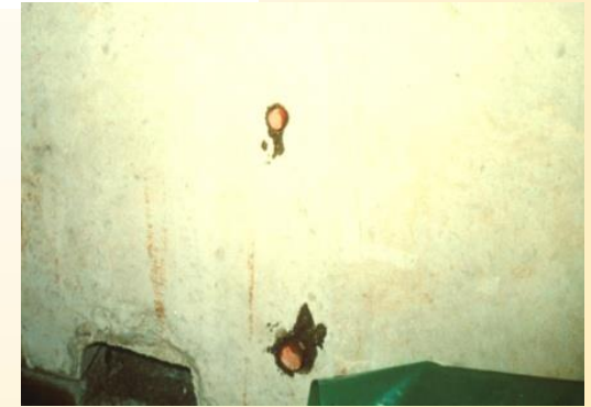
C: Withdraw the nozzle from the inlet hole and seal it with a rubber stopper.
