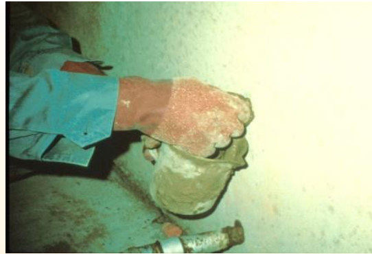
B: Catch the overflow in a cup and seal the outlet hole with a rubber stopper.
