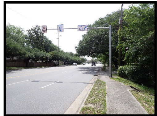
PHOTOGRAPH 2-04: MAST ARM SIGN STRUCTURE
