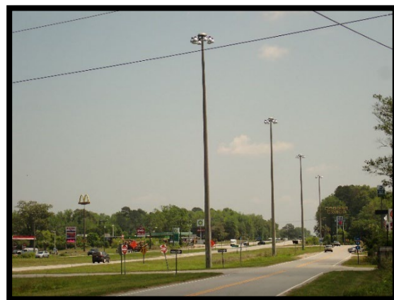
PHOTOGRAPH 3-24: HIGH MAST LIGHT POLE (CONCRETE)
