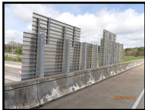
PHOTOGRAPH 3-18: BRIDGE MOUNTED (REAR)
