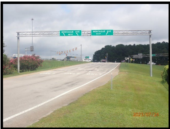
PHOTOGRAPH 3-09: 3-CHORD FULLSPAN (FRONT)
