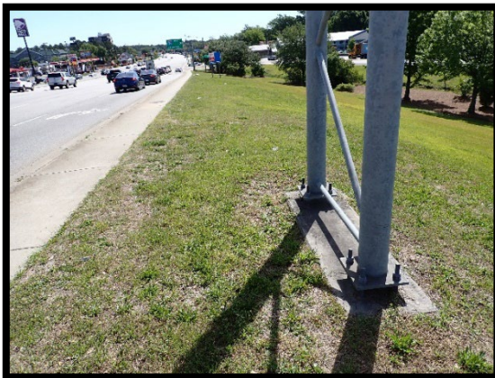
PHOTOGRAPH 1-09: FOUNDATION PHOTOGRAPH (MULTIPLE FOUNDATIONS)
