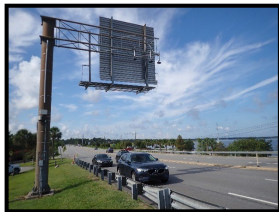
PHOTOGRAPH 3-06: 4-CHORD CANTILEVER (REAR)
