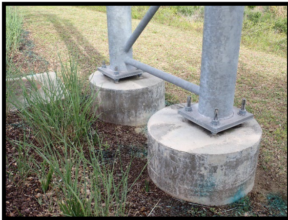
PHOTOGRAPH 3-27: TWO POST FRAME
