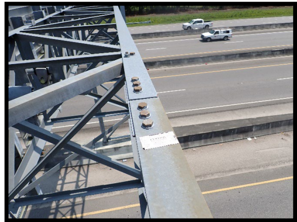
PHOTOGRAPH 4-11: TYPICAL BOX CHORD SPLICE
