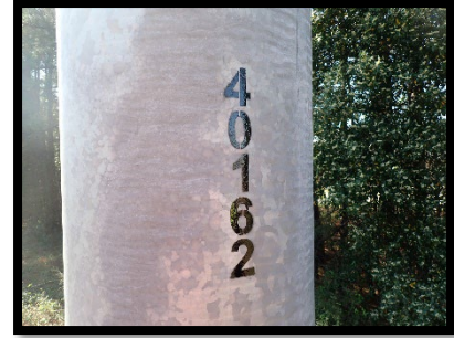
PHOTOGRAPH 2-06: STENCILING ON COLUMN
