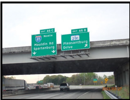
PHOTOGRAPH 3-17: BRIDGE MOUNTED (FRONT)
