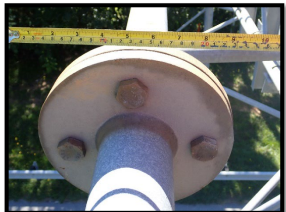
PHOTOGRAPH 1-12: TYPICAL SPLICE
