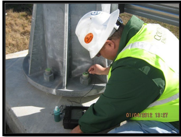
PHOTOGRAPH 1-14:4 INSPECTOR PERFORMING ULTRASONIC TEST
