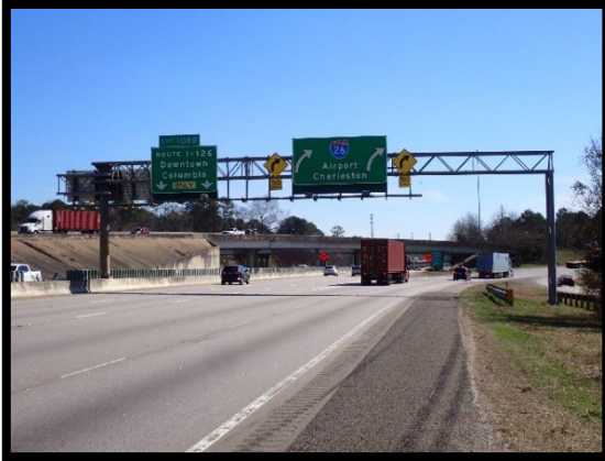
PHOTOGRAPH 3-13: 4-CHORD FULLSPAN WITH CANTILEVER (FRONT)
