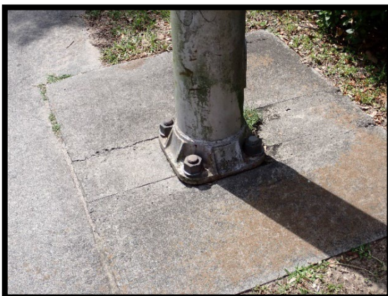
PHOTOGRAPH 1-11: FOUNDATION (SET IN SIDEWALK)
