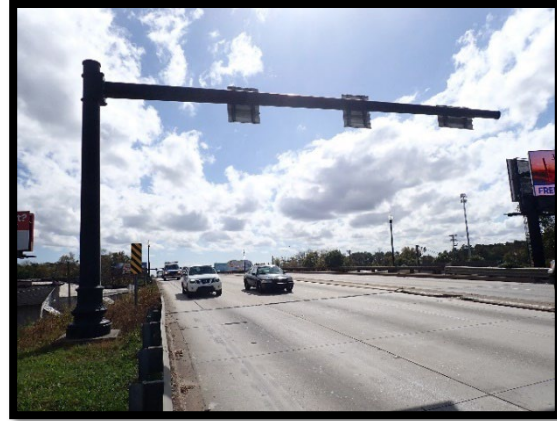
PHOTOGRAPH 3-20: MAST ARM (REAR)
