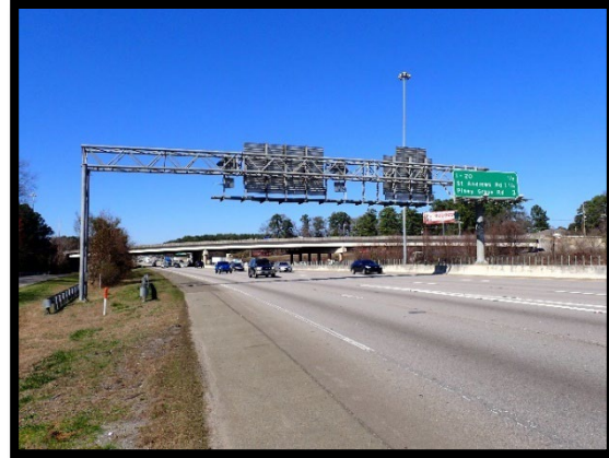
PHOTOGRAPH 3-14: 4-CHORD FULLSPAN WITH CANTILEVER (REAR)
