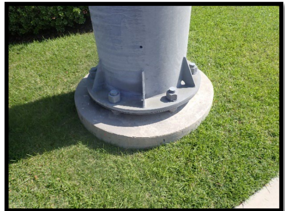
PHOTOGRAPH 1-10: FOUNDATION (SINGLE POST)
