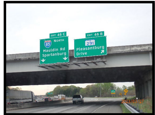
PHOTOGRAPH 2-03: BRIDGE MOUNTED SIGN STRUCTURE
