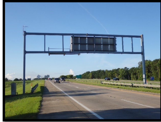
PHOTOGRAPH 3-08: 2-CHORD FULLSPAN (REAR)
