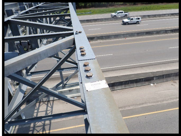
PHOTOGRAPH 3-34: BOX CHORD SPLICE
