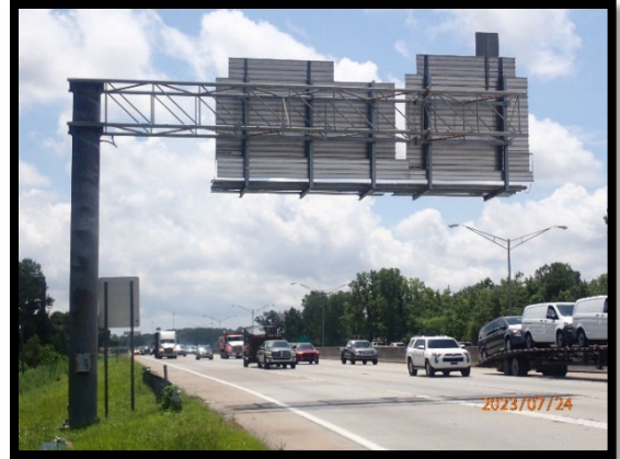
PHOTOGRAPH 1-08: OVERALL REAR PHOTOGRAPH
