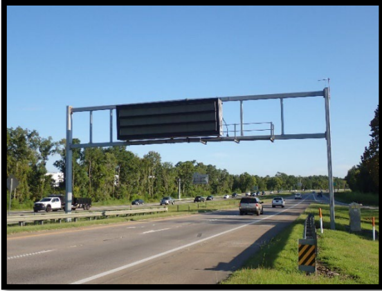
PHOTOGRAPH 3-07: 2-CHORD FULLSPAN (FRONT)
