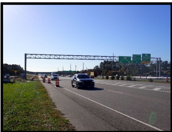
PHOTOGRAPH 3-11: 4-CHORD FULLSPAN (FRONT)
