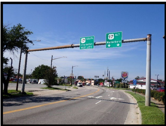
PHOTOGRAPH 3-21: MONOTUBE (FRONT)
