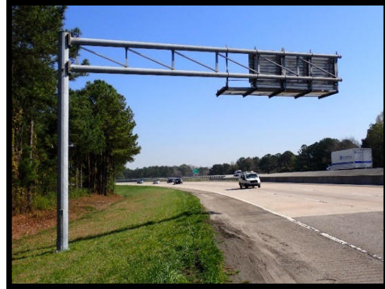
PHOTOGRAPH 3-02: 2-CHORD MAST ARM (REAR)
