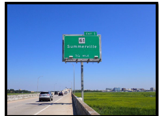
PHOTOGRAPH 2-02: BUTTERFLY SIGN STRUCTURE
