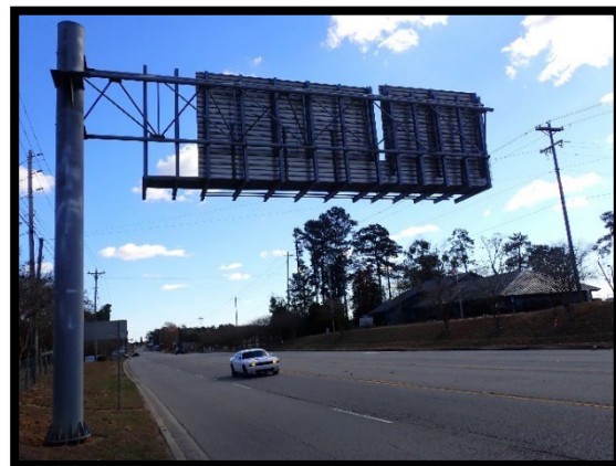
PHOTOGRAPH 3-04: 3-CHORD CANTILEVER (REAR)
