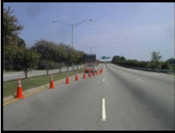
PHOTOGRAPH 1-05: STATIC LANE CLOSURE
