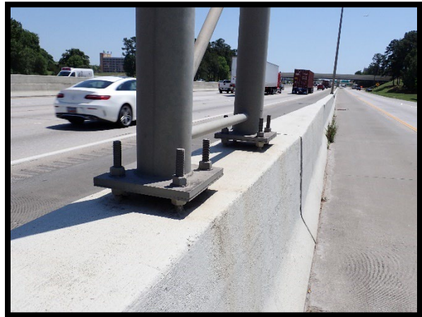
PHOTOGRAPH 3-30: GROUND MOUNTED (BARRIER FOUNDATION LISTED AS GROUND MOUNTED)
