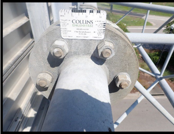
PHOTOGRAPH 3-33: ROUND CHORD SPLICE
