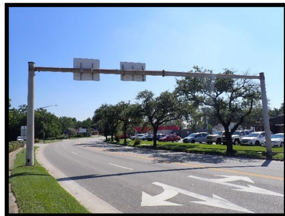
PHOTOGRAPH 3-22: MONOTUBE (REAR)
