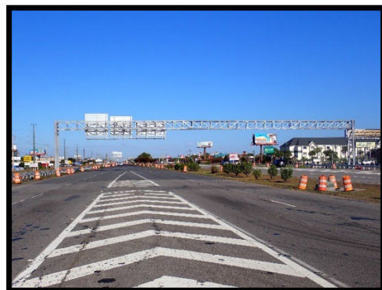
PHOTOGRAPH 3-12: 4-CHORD FULLSPAN (REAR)
