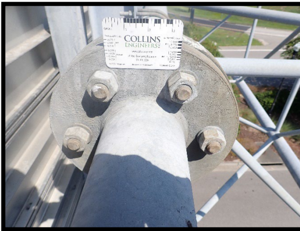
PHOTOGRAPH 4-10: TYPICAL ROUND SPLICE
