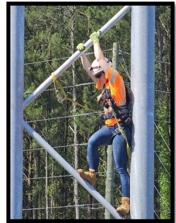
PHOTOGRAPH 1-01: INSPECTOR CLIMBING STRUCTURE
