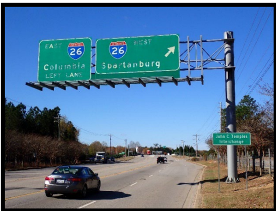
PHOTOGRAPH 3-03: 3-CHORD CANTILEVER (FRONT)
