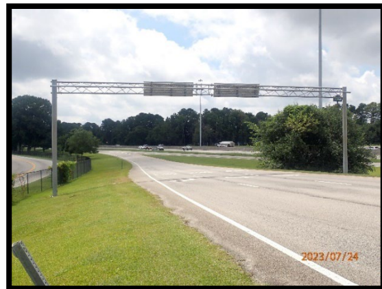
PHOTOGRAPH 3-10: 3-CHORD FULLSPAN (REAR)
