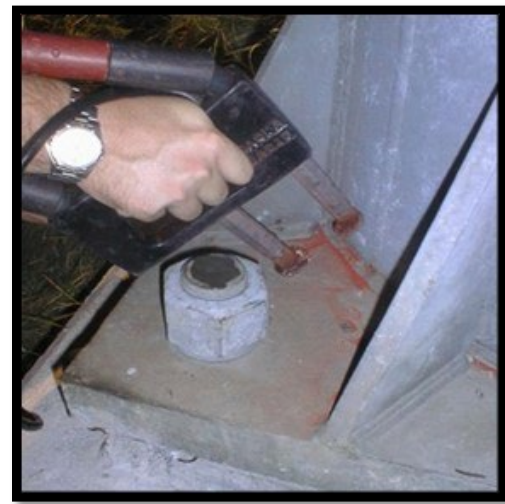
PHOTOGRAPH 1-15: INSPECTOR PERFORMING MAGNETIC PARTICLE TEST
