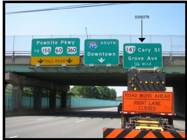
PHOTOGRAPH 1-06: MOBILE LANE CLOSURE
