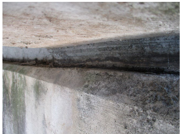
Photo 6. Non-ACM Bond Break Bearing Pad.
