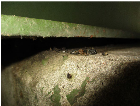
Photo 5. Non-ACM Bond Break Bearing Pad.
