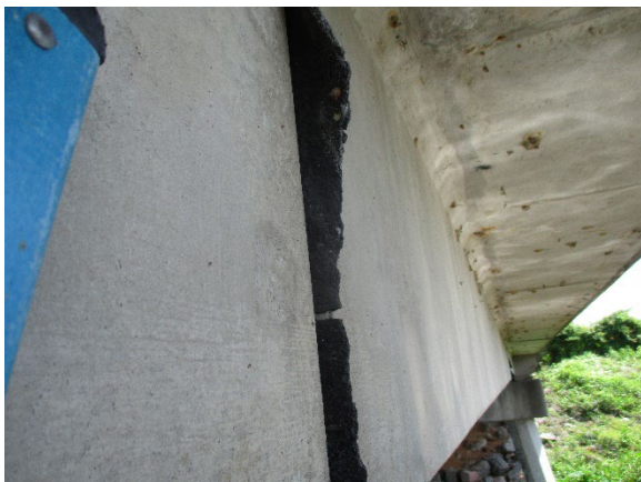
Photo 5. Non-ACM Expansion Joint Material.
