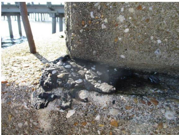
Photo 5. Non-ACM Expansion Joint Sealer.
