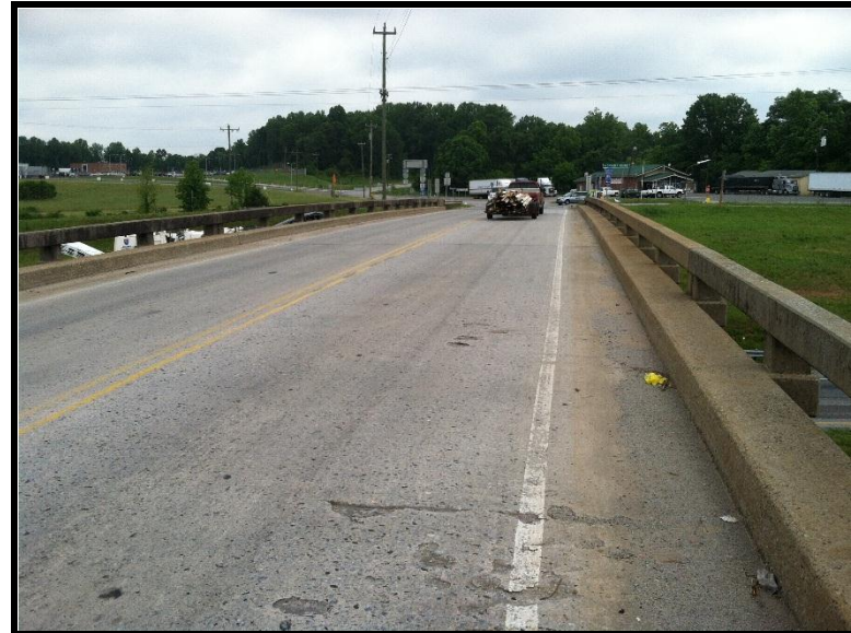
2 General view top deck Center line and lane boundary lines observed.
