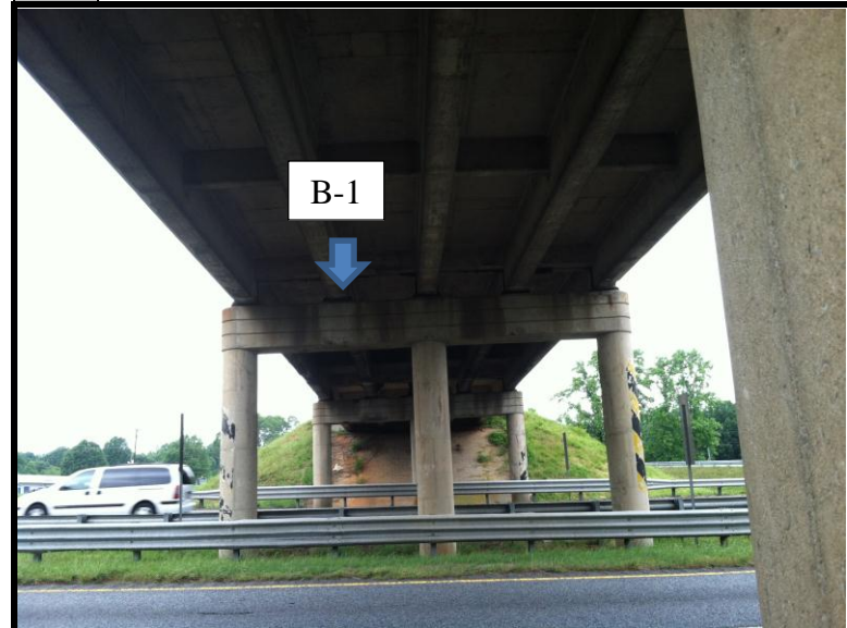
4 Asphalt expansion material located between deck panels. Sampled obtained from top of cross girder Sample B -
