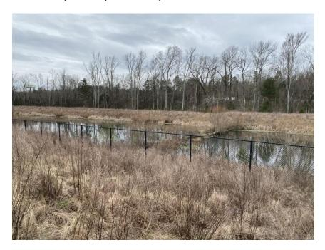
View of the existing pond and drainage structures impacted by the proposed right-ofway for the project. A portion of the existing pond at the northern end will be filled and the southern end of the pond expanded to provide for the volume lost.
