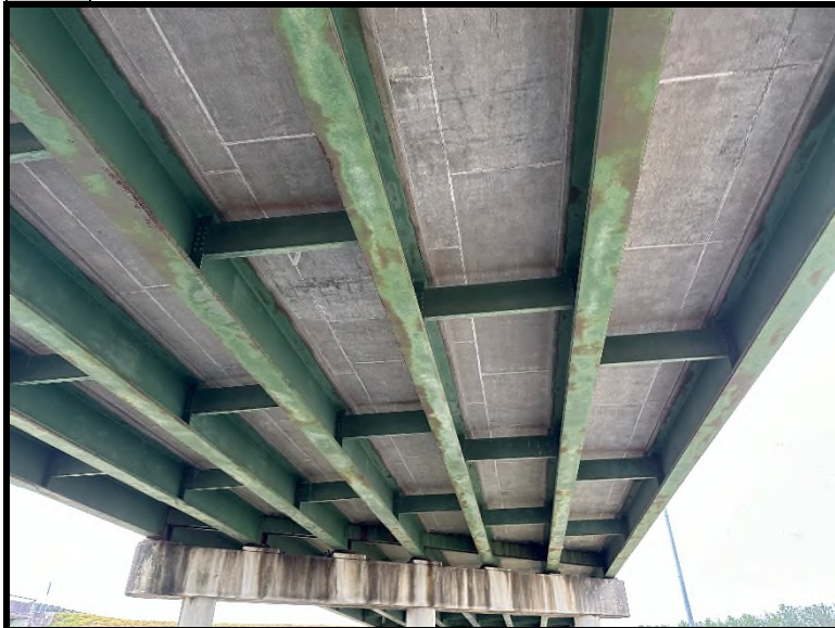
3 View beneath the bridge. The green structural steel tested positive for lead-based paint (5.9-6.4 mg/cm²).
