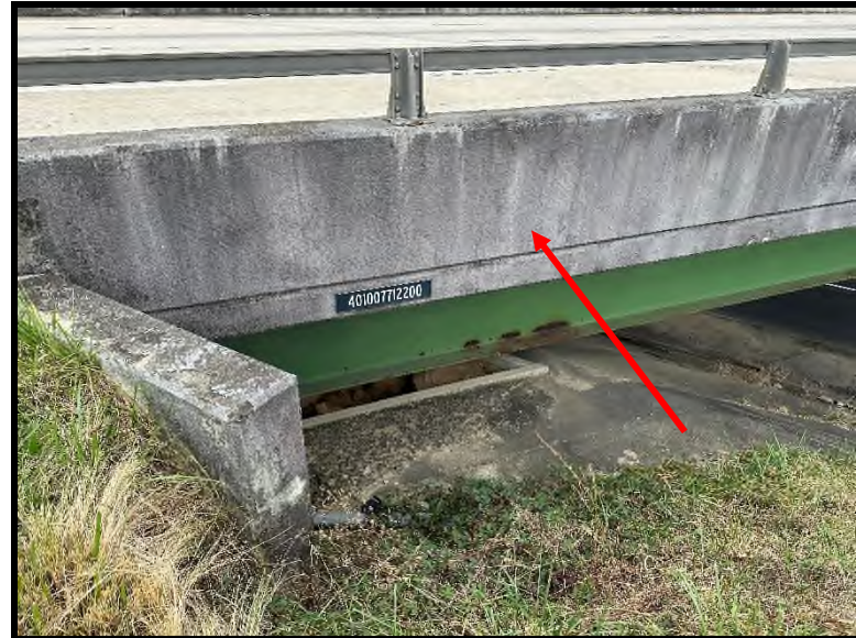
2 Structure number. The concrete surfacing texture tested positive for asbestos (2% Chrysotile).
