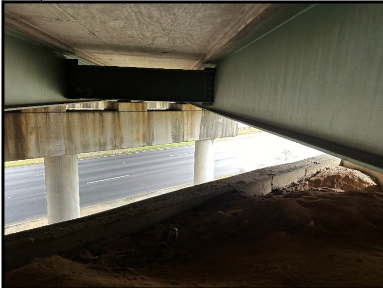
3 View beneath the bridge. The green structural steel tested positive for lead-based paint (6.6-7.6 mg/cm 2 ).
