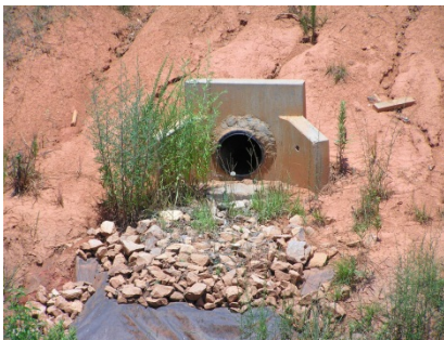
Use Pipe Flared End Section when specified in the plans or special provisions.
