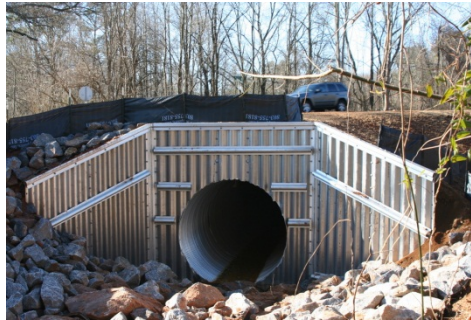
Use Pipe Flared End Section when specified in the plans or special provisions.
