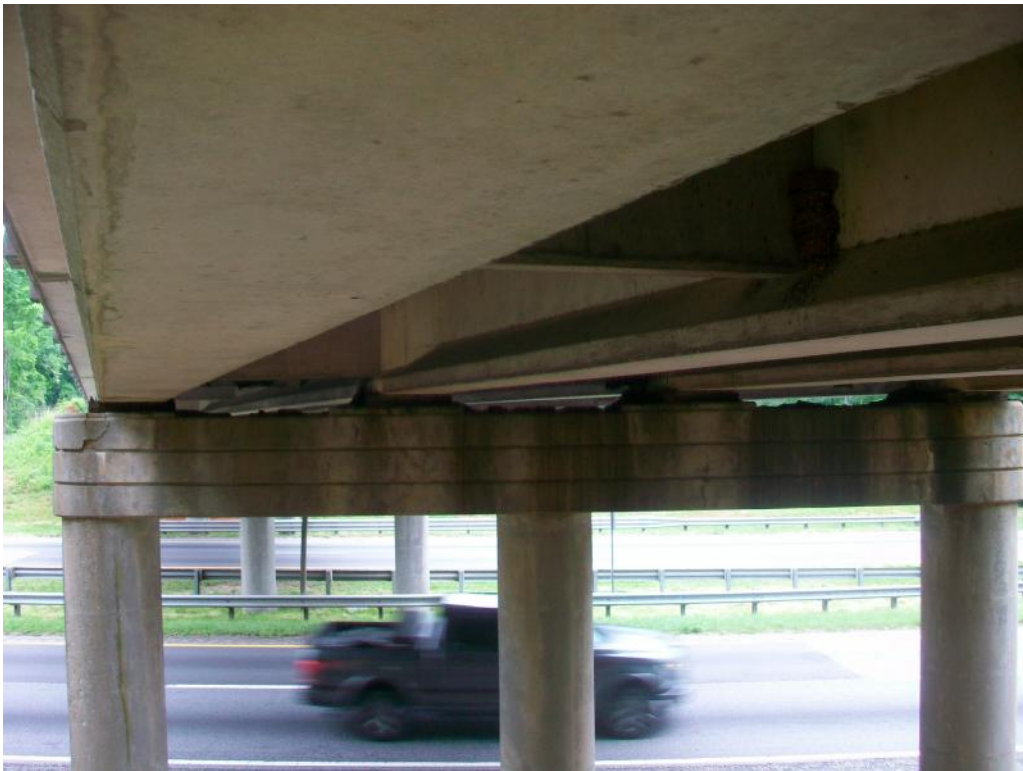
Photograph 4 – View of the underside of the bridge. All metal bridge components, except for the galvanized metal guardrails are coated with lead based paint.
