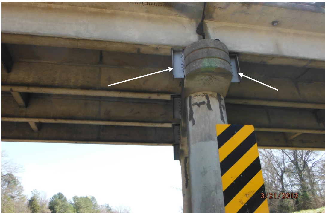
Pieces of I-Beam anchored to bent cap to support beam
