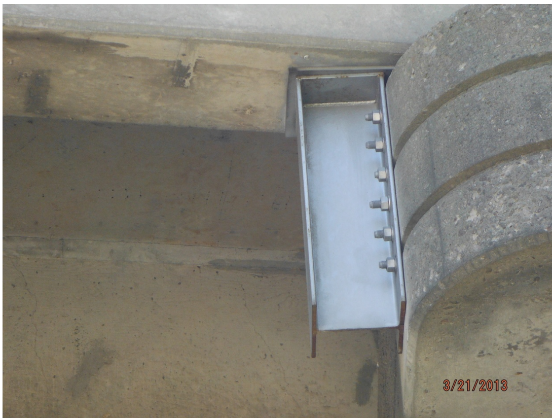
Pieces of I-Beam anchored to bent cap to support beam
