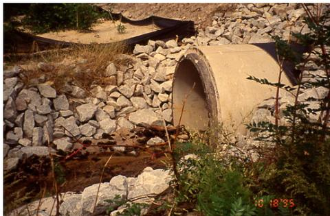
For all exposed crossline pipe ends, when an end treatment is not specified in the plans, use **Pipe Riprap Protection** (804-3xx-xx). For flexible pipe larger than 24" diameter, install pipe straight headwall, pipe end structure, flared end
