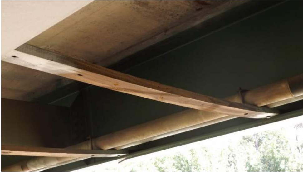
Figure 14 – Wooden Slats supporting Conduit
