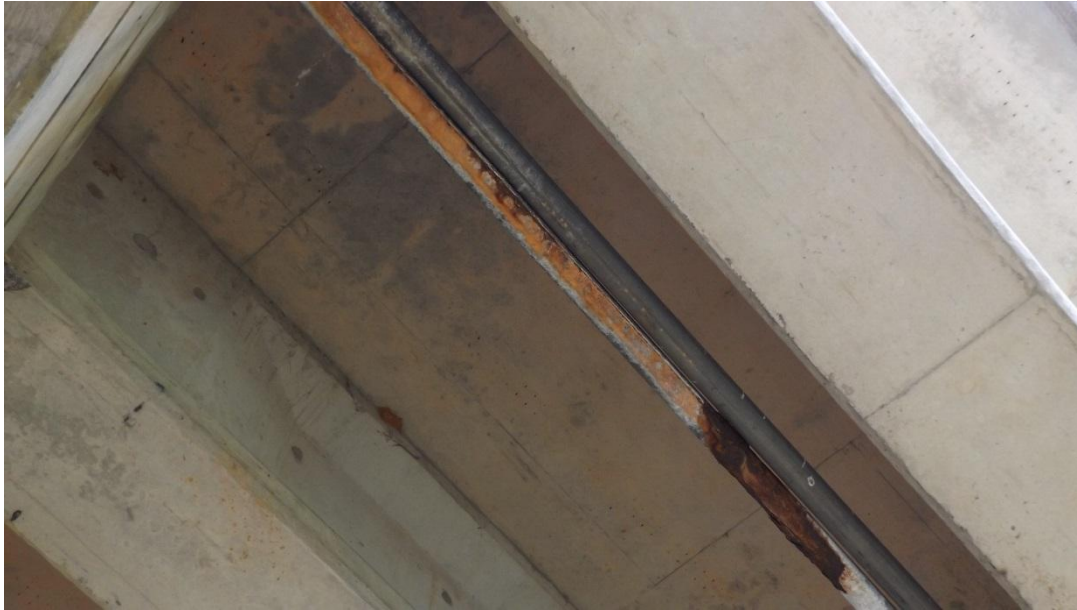
Figure 14 – Conduit Corrosion
