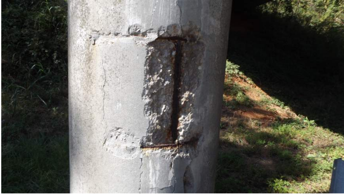
Figure 11 - Spall on Column
