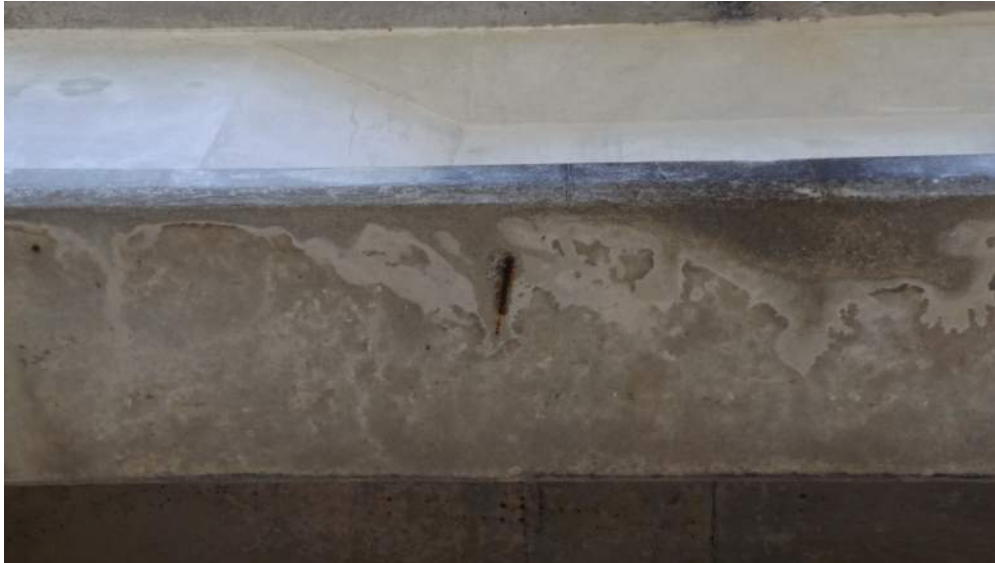
Figure 4 – Exposed Rebar in Beam
