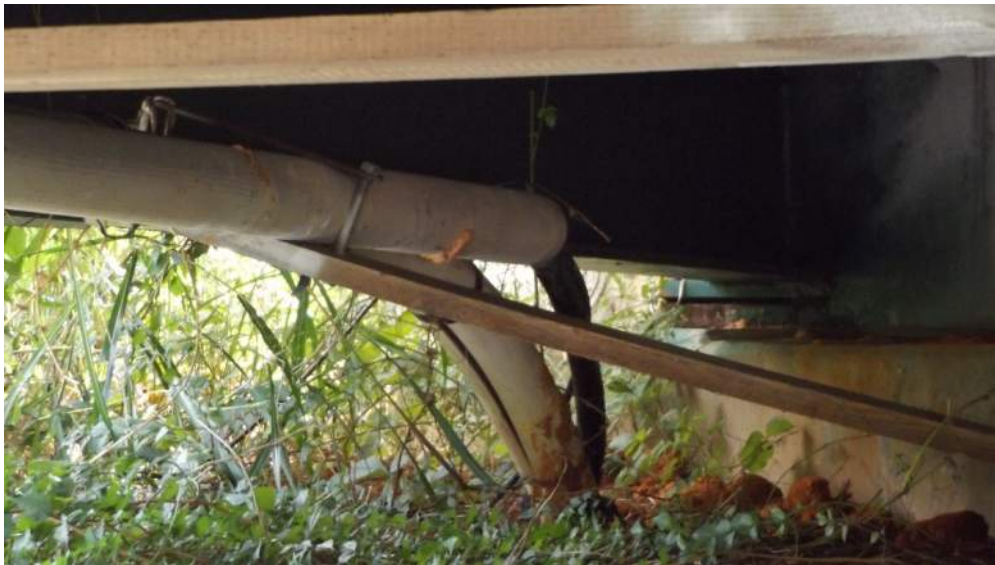
Figure 15 – Wooden Slat has fallen off the Beam
