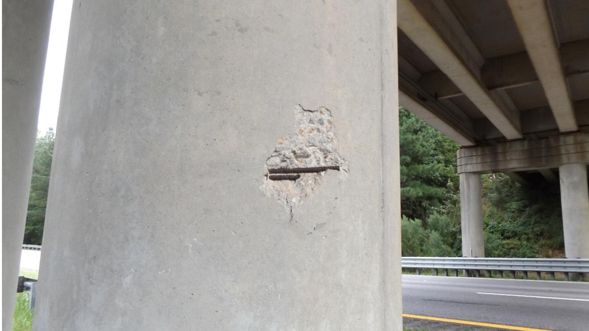
Figure 12 – Spall in Column
