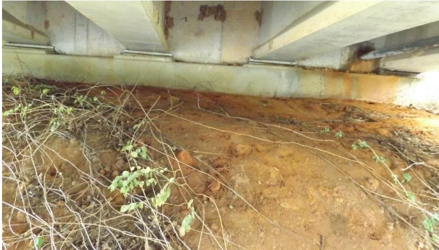
Figure 6 – End Bent Bearings
