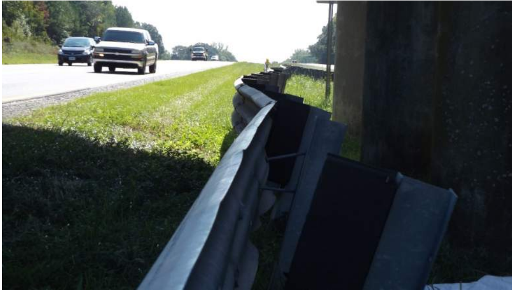
Figure 13 – Guardrail Damage
