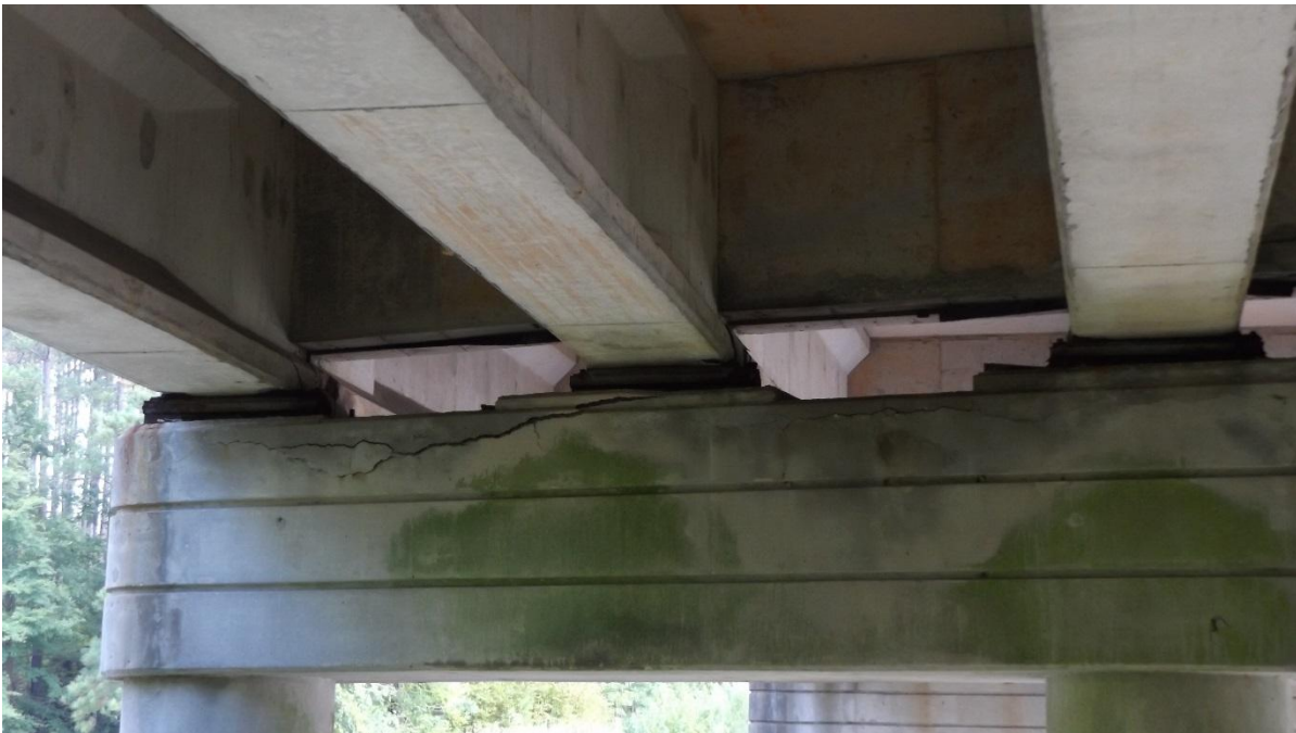
Figure 11 – Horizontal Crack in Bent Cap
