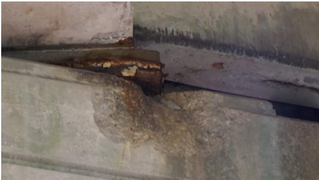
Figure 10 - Spall on Top of Pier Cap
