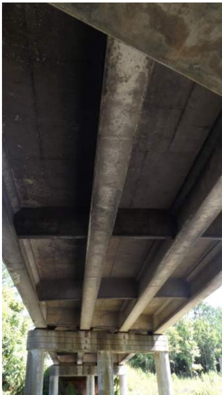
Figure 5 – Superstructure (from underneath) and Collision Damage to Bottom of Beam
