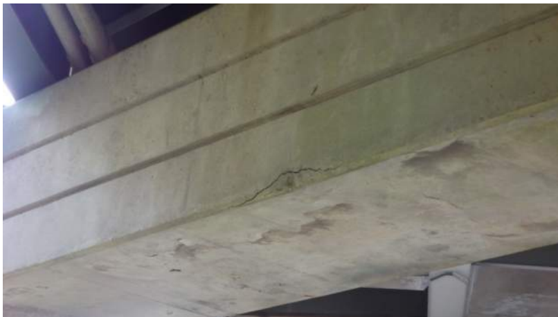
Figure 10 – Crack in Interior Bent Cap
