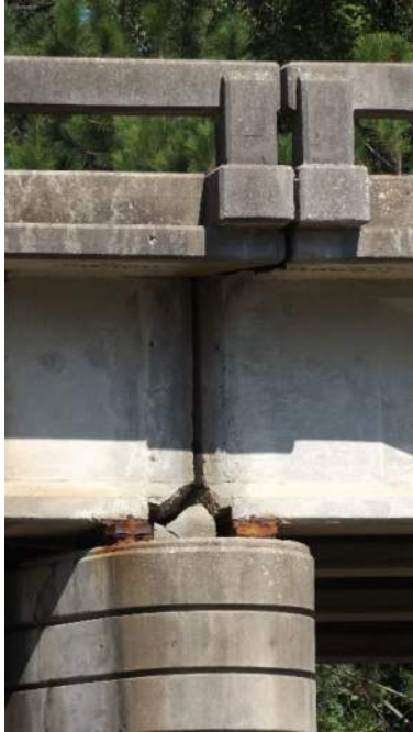
Figure 6 – Portion of End Diaphragm cracked off
