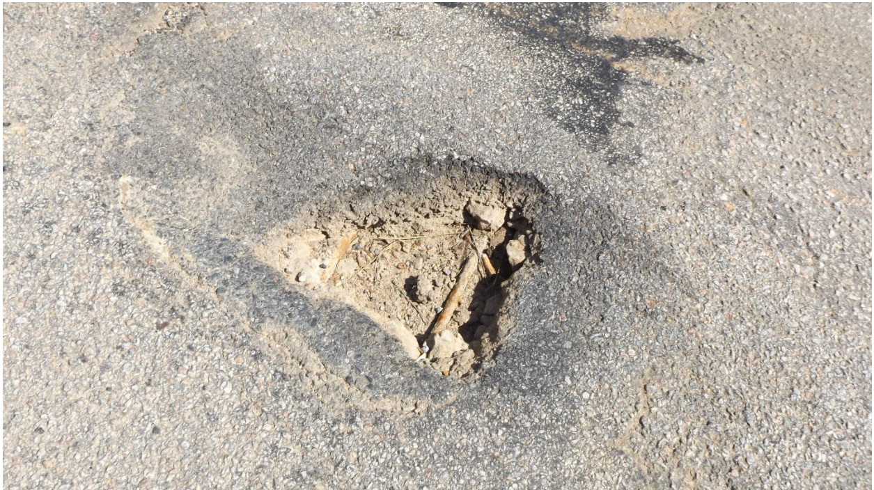
Figure 5 – Exposed Rebar in Concrete Deck
