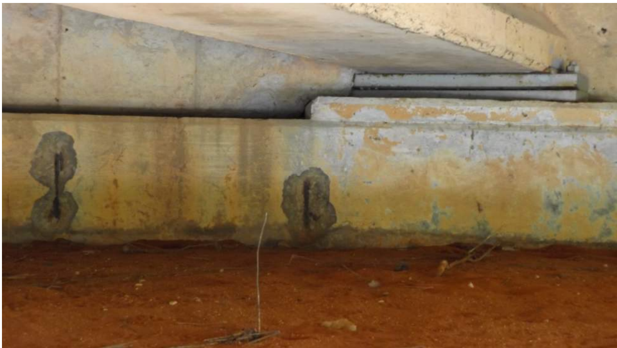
Figure 12 - End Bent Spalling
