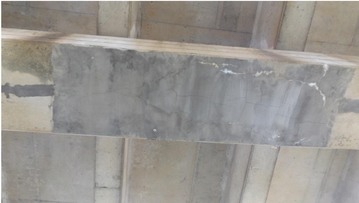
Figure 8 – Repaired Area in Cap
