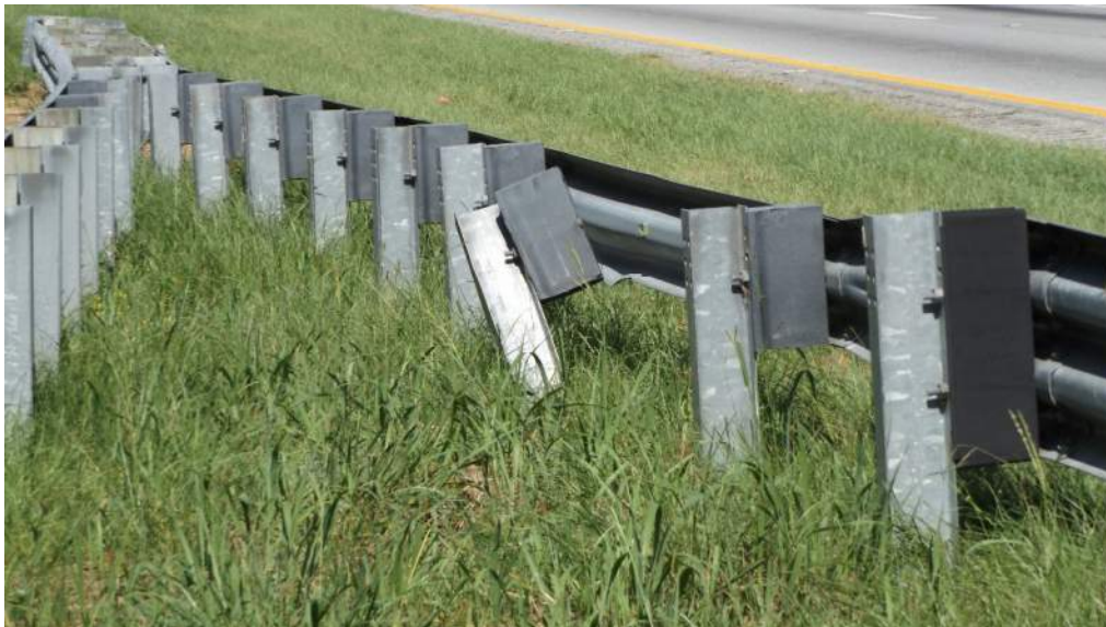
Figure 14 – Guardrail Damage
