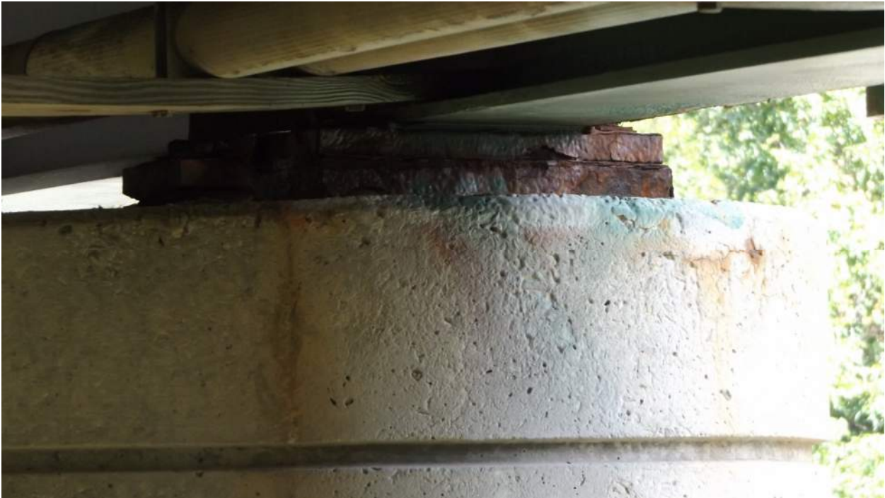
Figure 8 – Interior Bent Bearing
