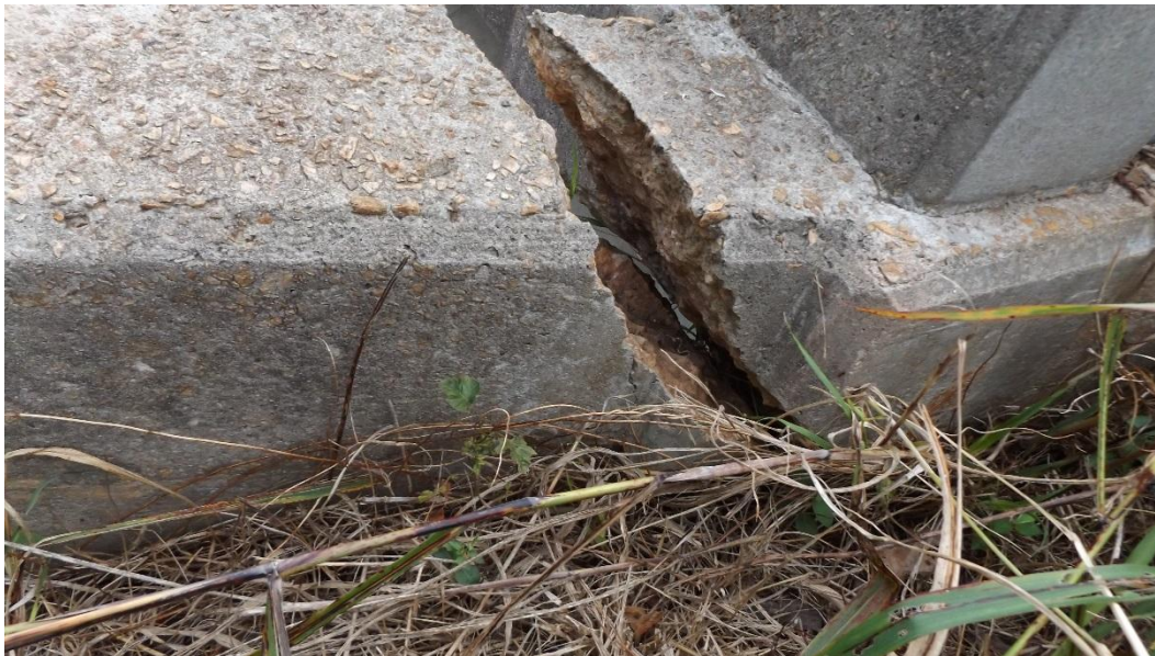
Figure 13 – Crack in Wing Wall
