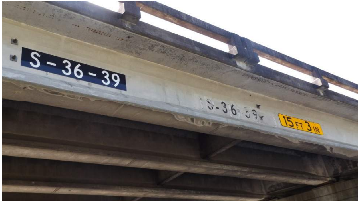
Figure 15 - Vertical Clearance
