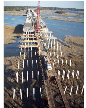
Trestle access successfully deployed to construct the Truman Parkway twin bridges over the Vernon River in Savannah, Georgia.
