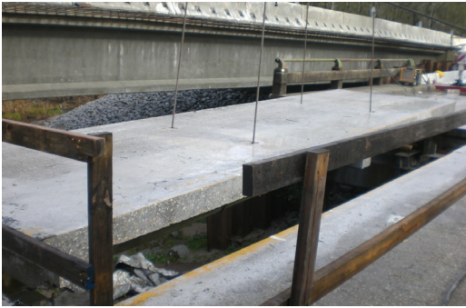
Balfour Beatty successfully removed deck sections on the SC 917 project for recycling.
