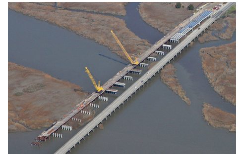
Balfour Beatty has worked around limited access and live traffic while building access trestle and foundation to a new crossing (Back River Bridge, Savannah, Georgia).
