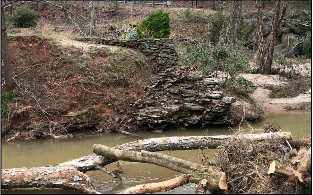
Figure 14. View of Eastern Section of Dam, Facing Southeast.
