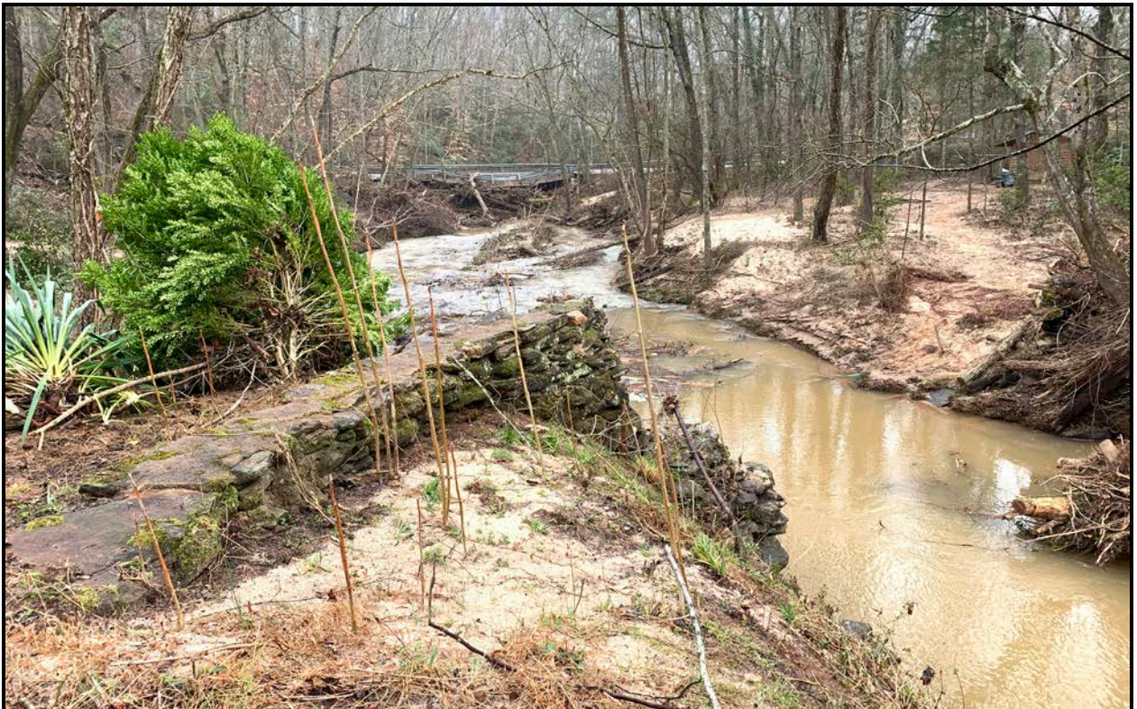
Figure 15. View of Eastern Section of Dam, Facing South.
