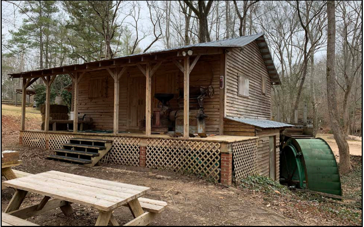
Figure 28. View of Timms Mill Main Building (3509.01), Facing Northeast from Creek.
