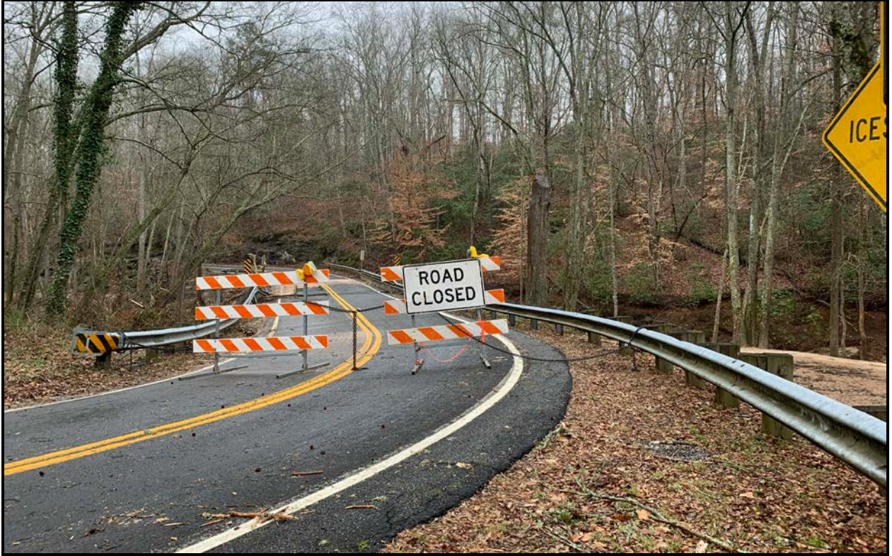
Figure 4. View of Project Area from West Side of Bridge, Facing East.
