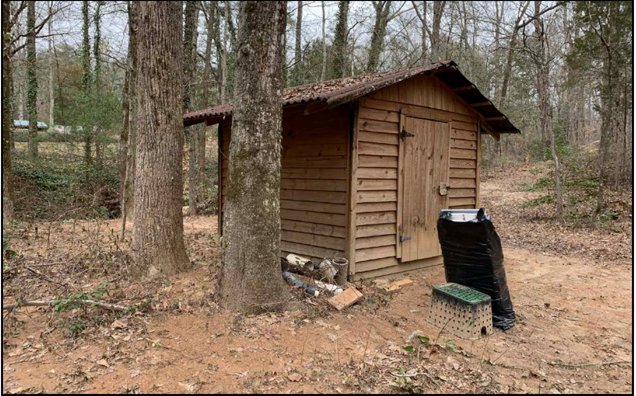
Figure 34. View of Current Pumphouse that Supplies the Mill with Water, Facing Northwest.
