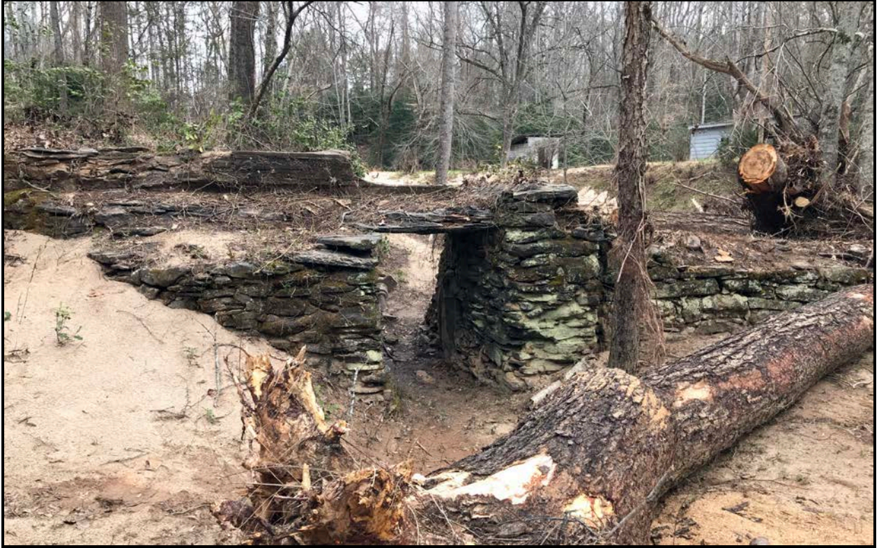
Figure 12. View of Western Portion of Dam, Facing Northeast.
