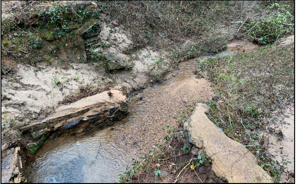
Figure 18. View of Mill Race Dam, Facing East.
