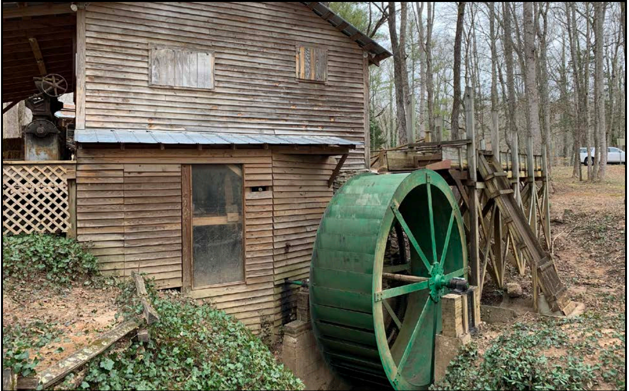
Figure 29. View of Timms Mill Main Building (3509.01), Facing North.
