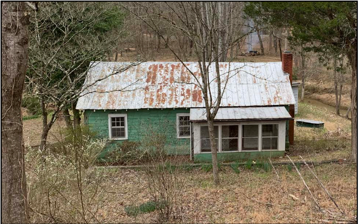
Figure 39. View of Resource 3509.07, Facing Northwest.
