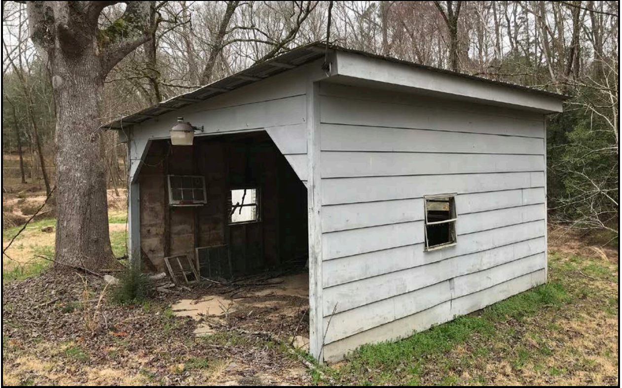
Figure 44. View of Resource 3509.11, Facing Northwest.
