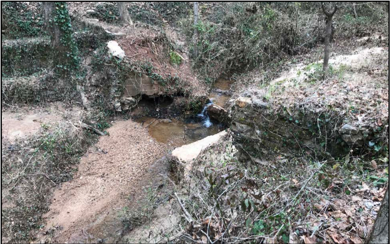
Figure 19. View of Mill Race Dam, Facing Northwest.
