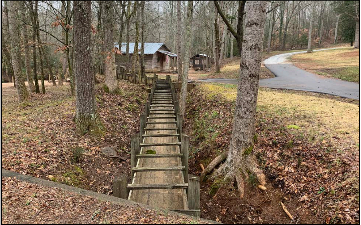
Figure 38. View of Rebuilt Flume in Original Mill Race, View from Above Culvert, Facing West.
