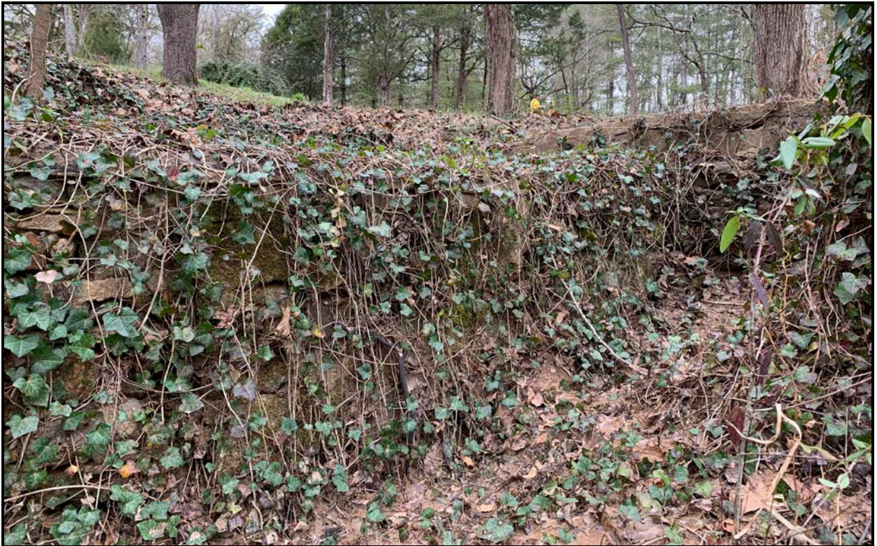
Figure 17. View of Exterior (Eastern) Wall of Mill Race, Facing Northwest.
