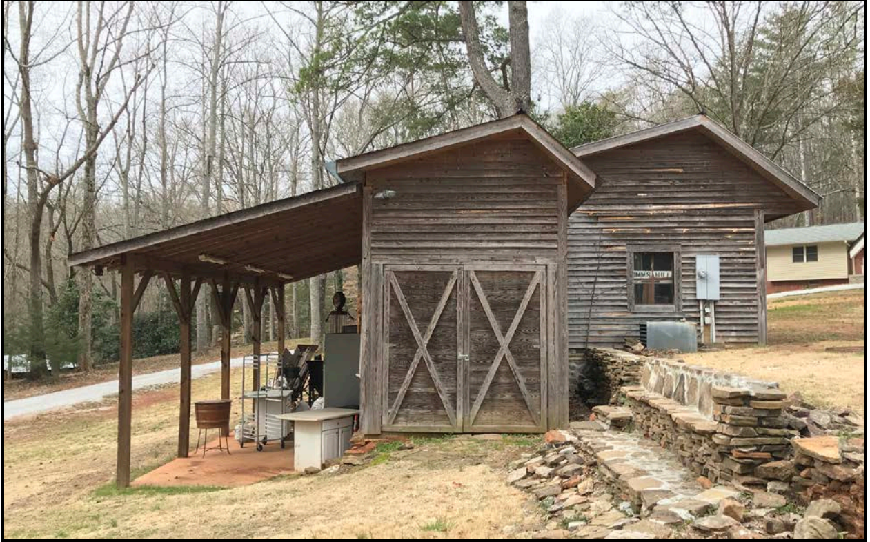
Figure 32. View of Timms Mill Country Store (3509.02), Facing West.
