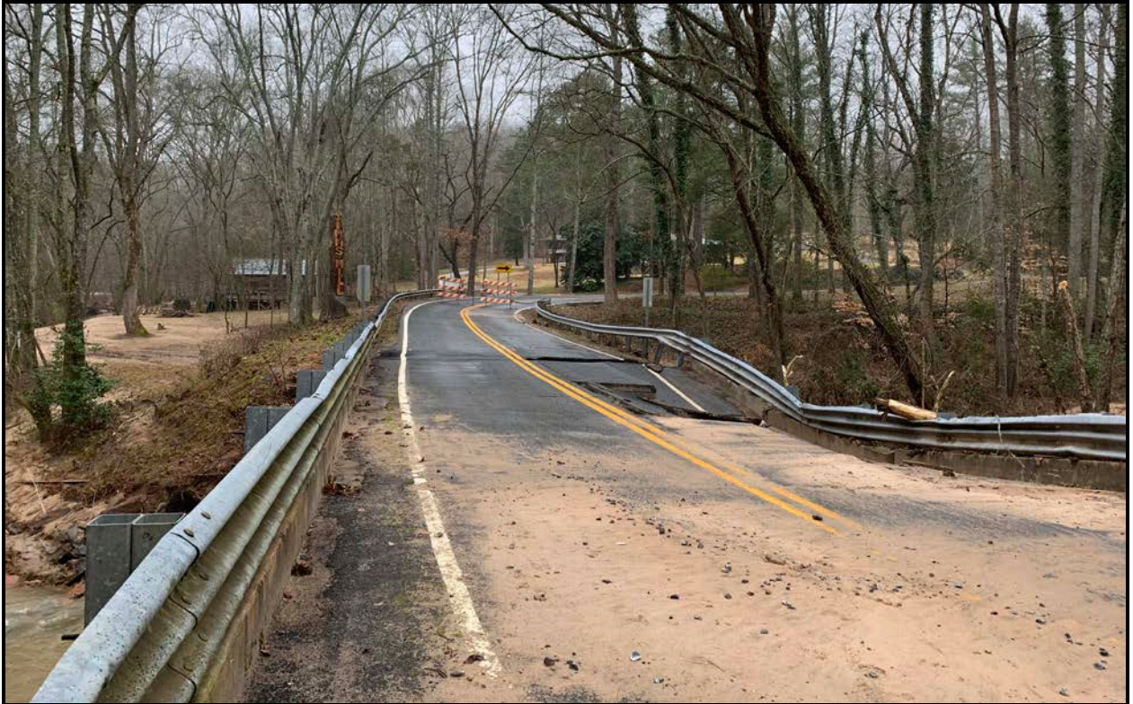
Figure 5. View of Project Area from East Side of Bridge, Facing West.
