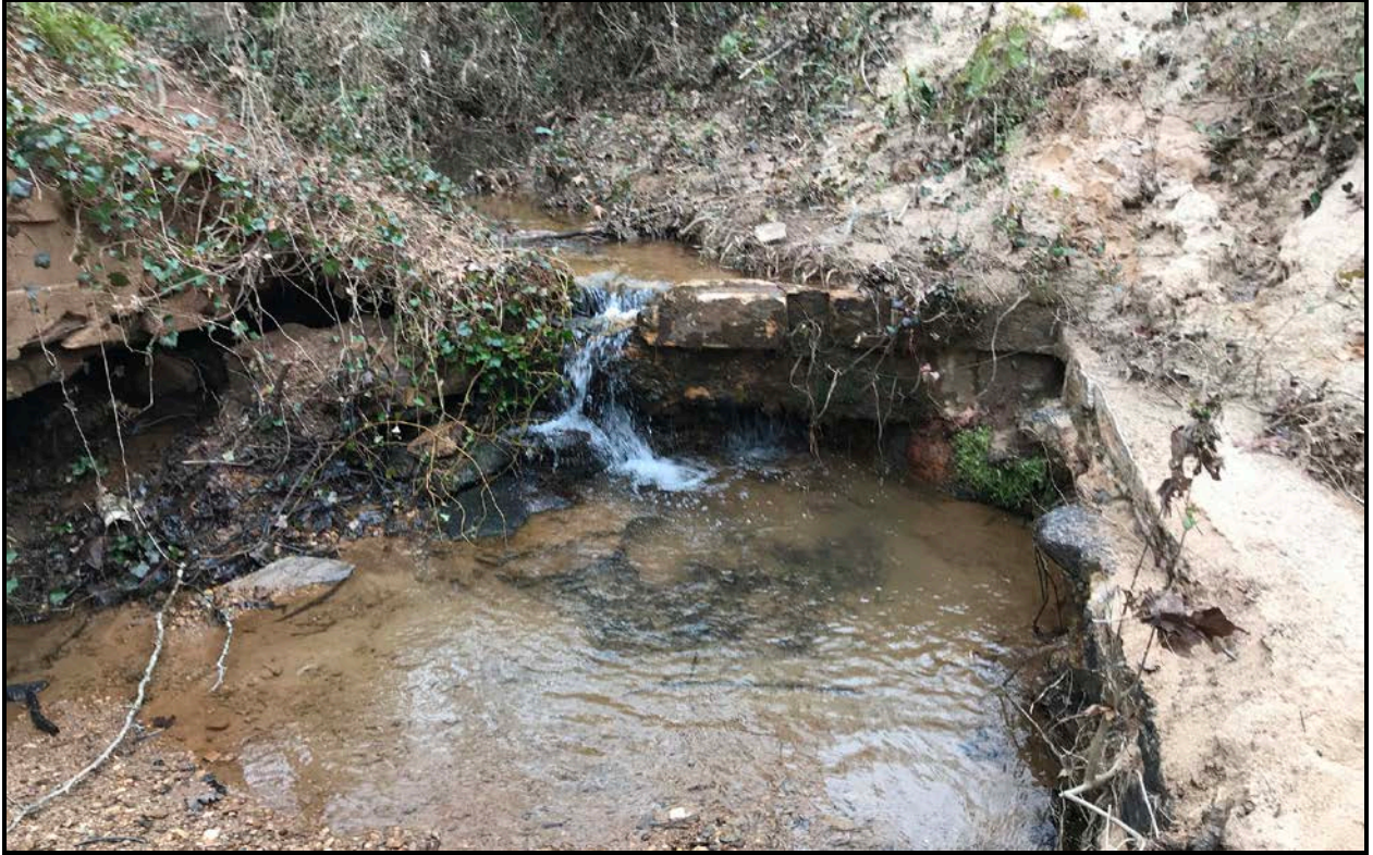
Figure 20. View of Mill Race Dam, Facing North.
