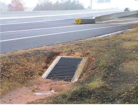
Use **Pipe End Structure** (719-615-00) when specified in the plans or special provisions. Use pipe end structure in locations where pipe exposed end faces the direction of traffic. Pipe end structures may be used in other locations if approved by the RCE.
