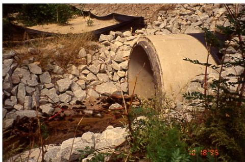
For all exposed crossline pipe ends, when an end treatment is not specified in the plans, use **Pipe Riprap Protection** (804-3xx-xx). For flexible pipe larger than 24" diameter, install pipe straight headwall, pipe end structure, flared end section, or wingwall section in addition to riprap. For all exposed driveway pipe ends where no end treatment
