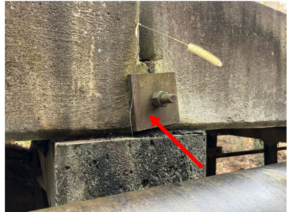
Photo 4. LBP on Orange Tie Rod Washer.
