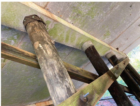
Photo 5. End Cap Support Underside View.
