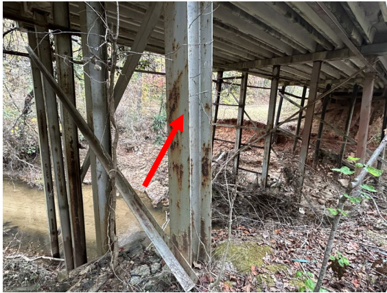
Photo 3. Underside View of Bridge and Silver LBP on Steel Structural Support.
