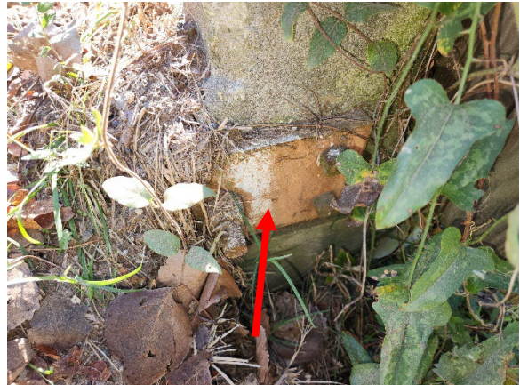
Photo 4. LBP on Rust Colored Tie-Rod Washer.
