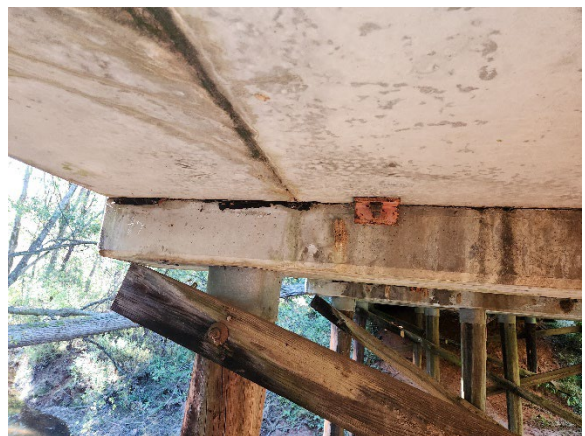
Photo 6. Non-ACM Bent Cap Bearing Pad.
