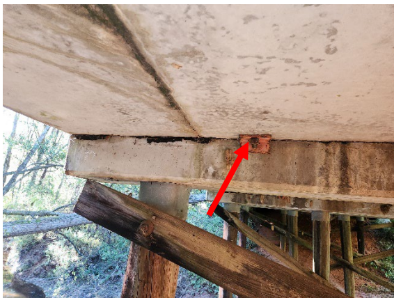
Photo 5. LBP on Orange/Rust L-Bracket.
