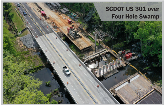
On US 301 over Four Hole Swamp, Crowder utilized a trestle to access interior piles. Our team will use the same method for Package 27's SC-83 bridge construction.
