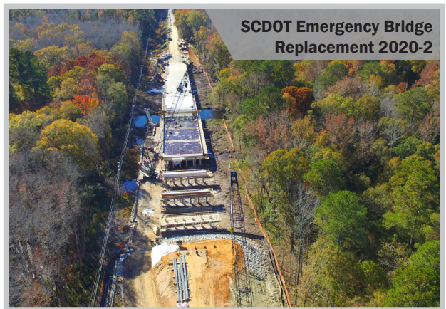
Crowder constructed two types of superstructures for the SC-4 over South Edisto River 610' 3-span bridge. The 250'+ approach spans utilized a 40' long span flat slabs system, and for over the main 90' channel, the team used a more traditional approach with type III precast girders and an 8" cast in place deck.
