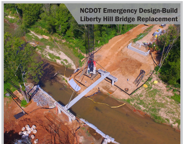
Crowder replaced a 240' long bridge with a 270' long structure in Mooreville, NC. This three-span structure was founded on four each 36" diameter drilled shaft at the two interior bents and H Pile end bents. The superstructure consisted of 39" Box Beams, 540 LF of cast in place barrier rail, and an asphalt overlay.
