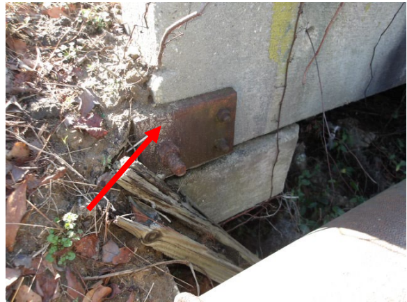
Photo 2. LBP on Tie-Rod Washer on Both Sides of the Bridge.
