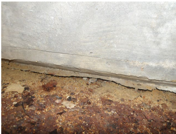
Photo 3. Non-ACM Cementitious Bond Break Material.
