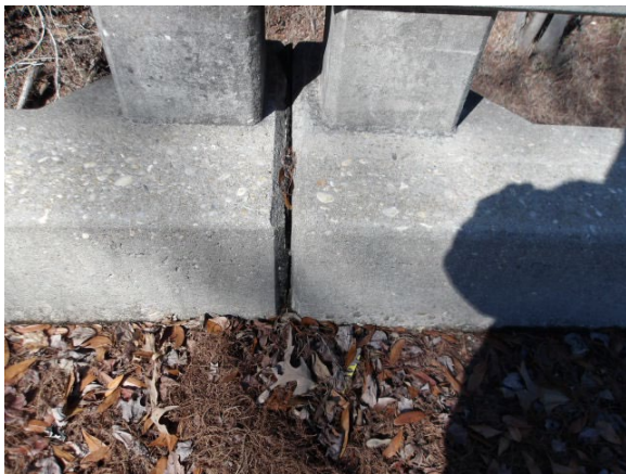
Photo 5. Non-ACM Expansion Joint Material.
