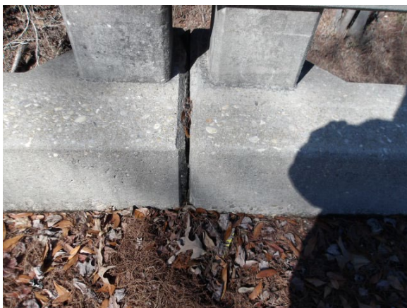
Photo 5. Non-ACM Expansion Joint Material.
