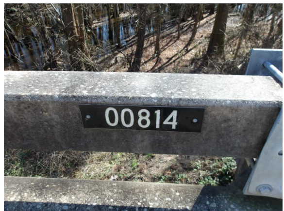
Photo 6. SCDOT Bridge Asset # Attached to the Concrete Guardrail.
