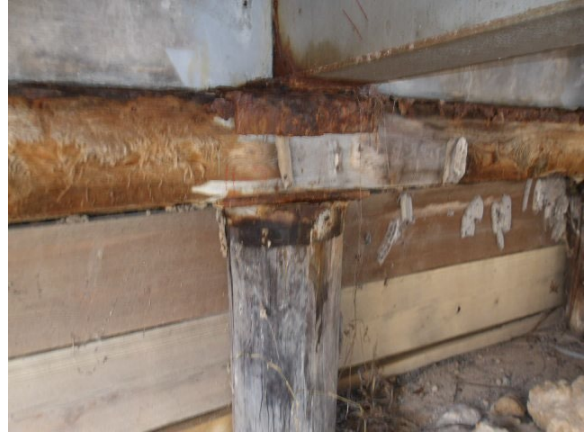
Photo 2. Non-ACM Timber Pile Cap Felt.
