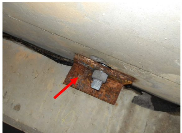
Photo 4. LBP on L-Brackets on Underside of Bridge.
