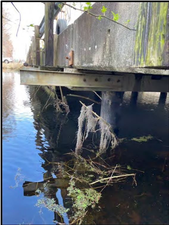
Looking Northeast, Pile Header
