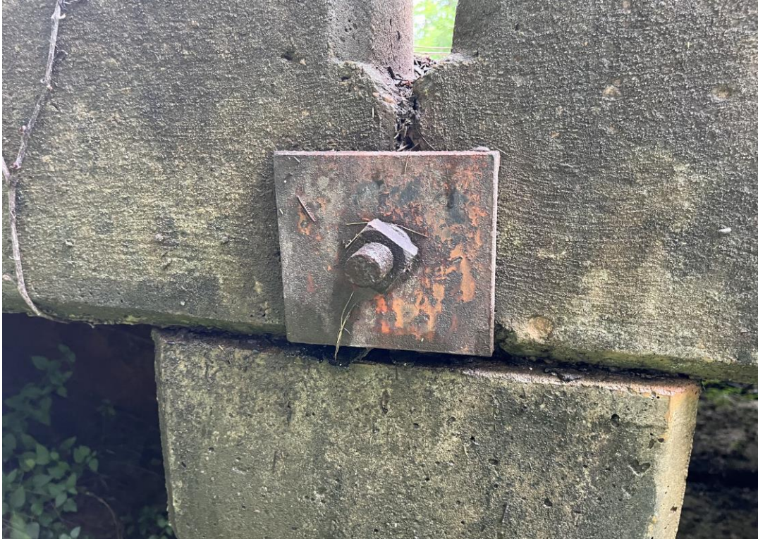
Photo 5 View of corroded orange metal bracket.
