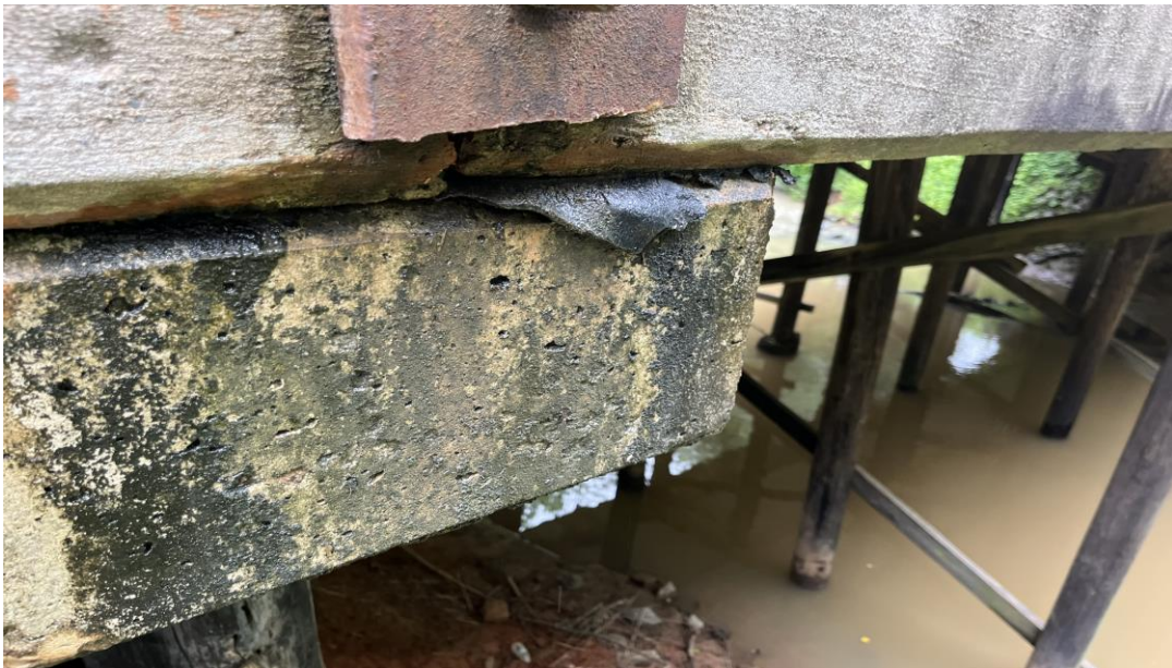
Photo 6 View of thick friction barrier between pier and pier cap
