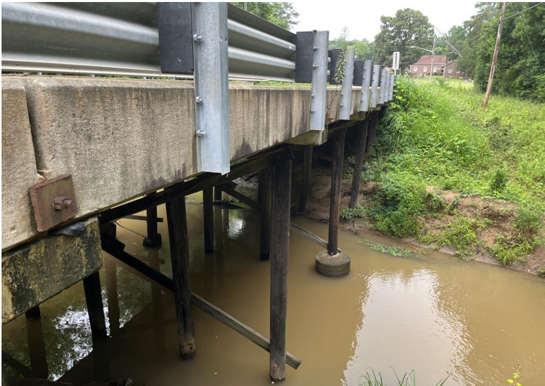
Photo 4 View of the side of the bridge to the west with the metal brackets on the side.
