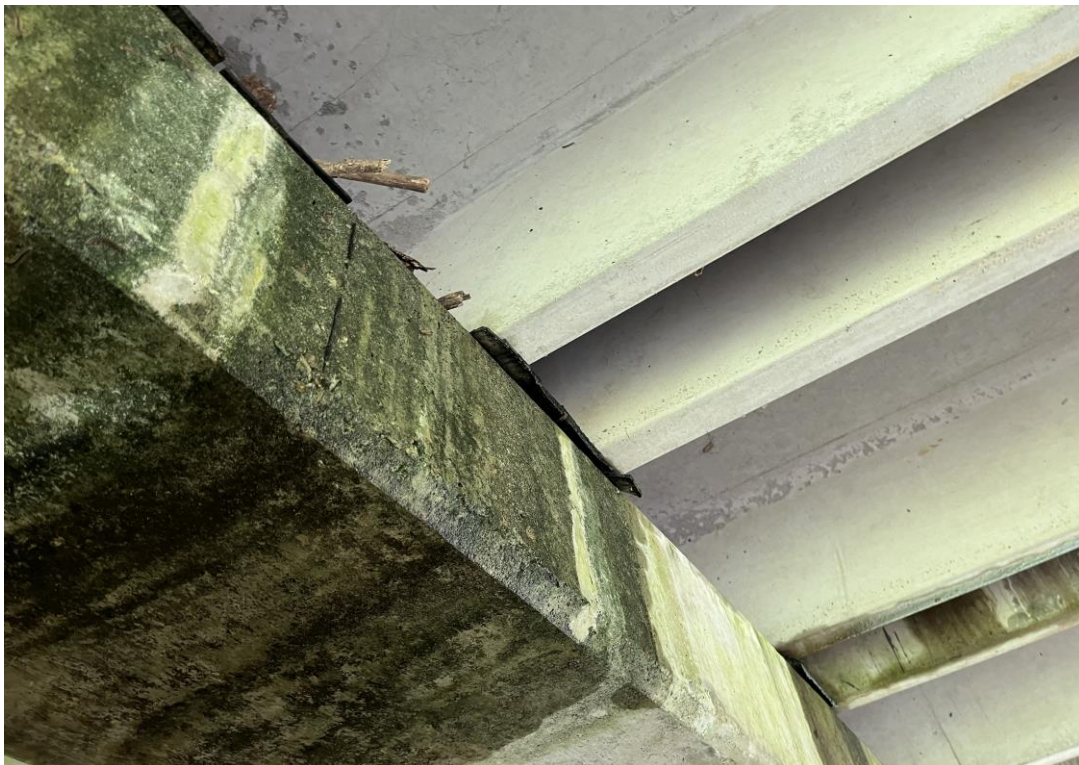
Photo 4 View of thick friction barrier between pier cap and decking.
