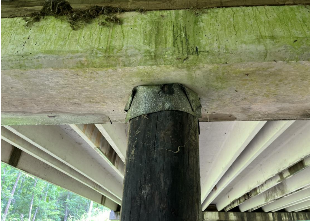
Photo 3 View of thin friction barrier between pier and pier cap.
