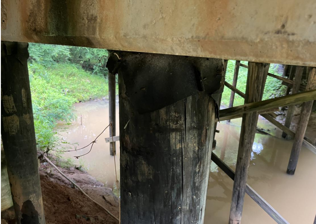
Photo 5 View of thin friction barrier between pier and pier cap.
