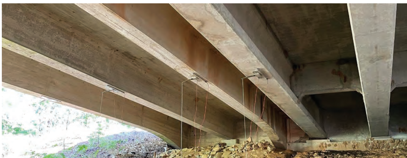
Figure 14: Installed Instrumentation - BR 568
