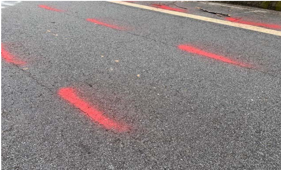
Reflective Cracking: Moderate - DF = 0.35 Lane
