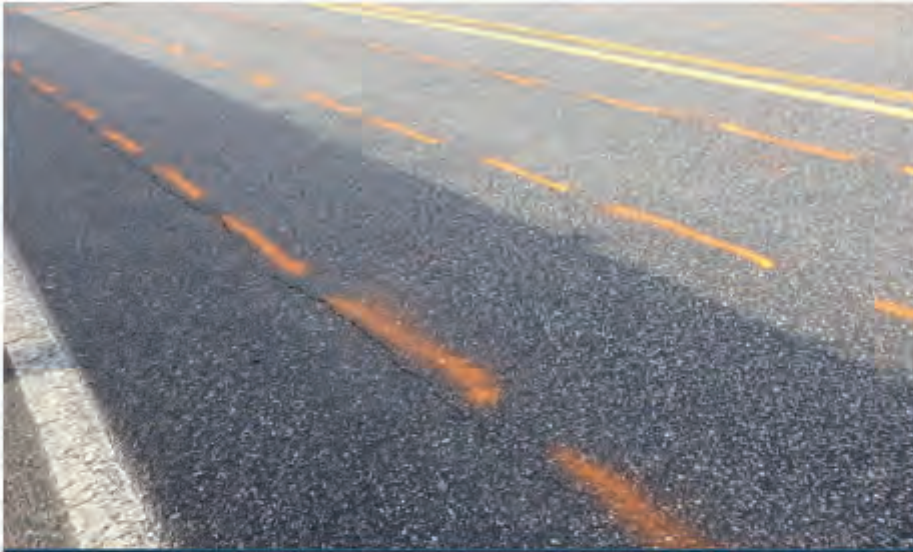
Reflective Cracking: Moderate - DF = 0.35 Lane
