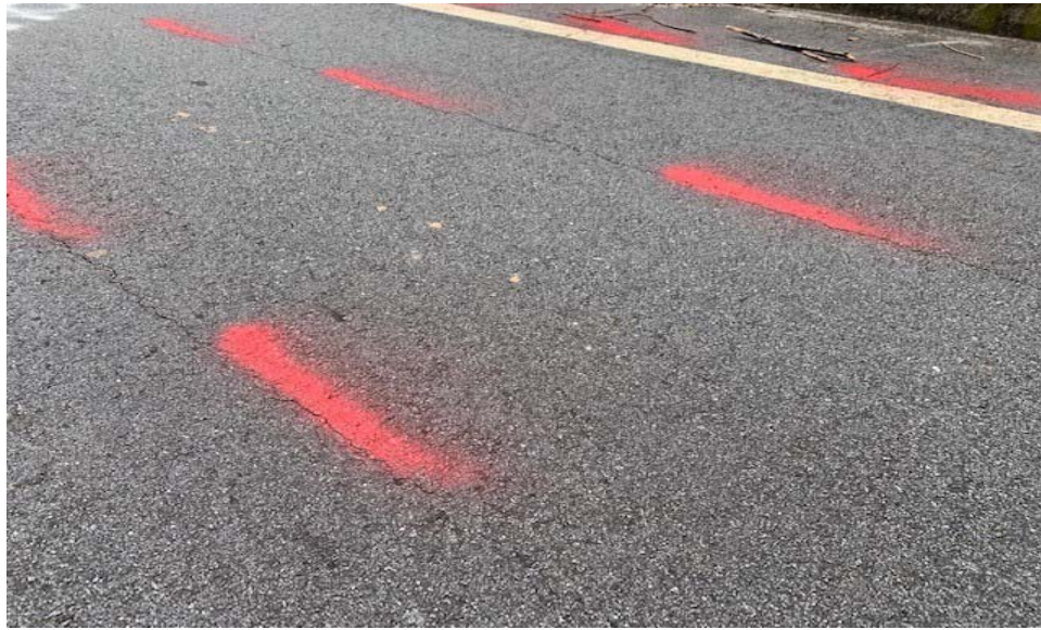
Figure 3 Bridge Deck Asphalt Overlay; Moderate Reflective Cracking
