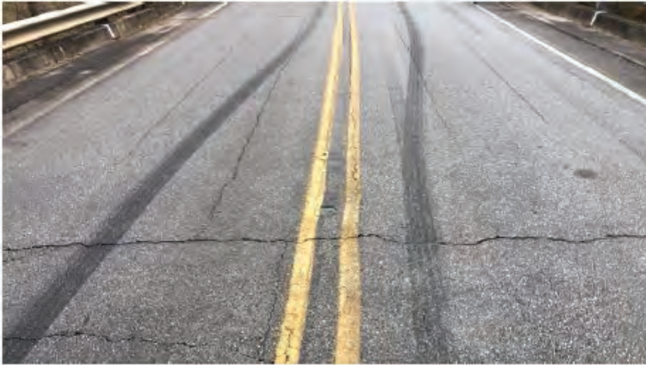
Reflective Cracking: Severe - DF = 0.5 Lane
