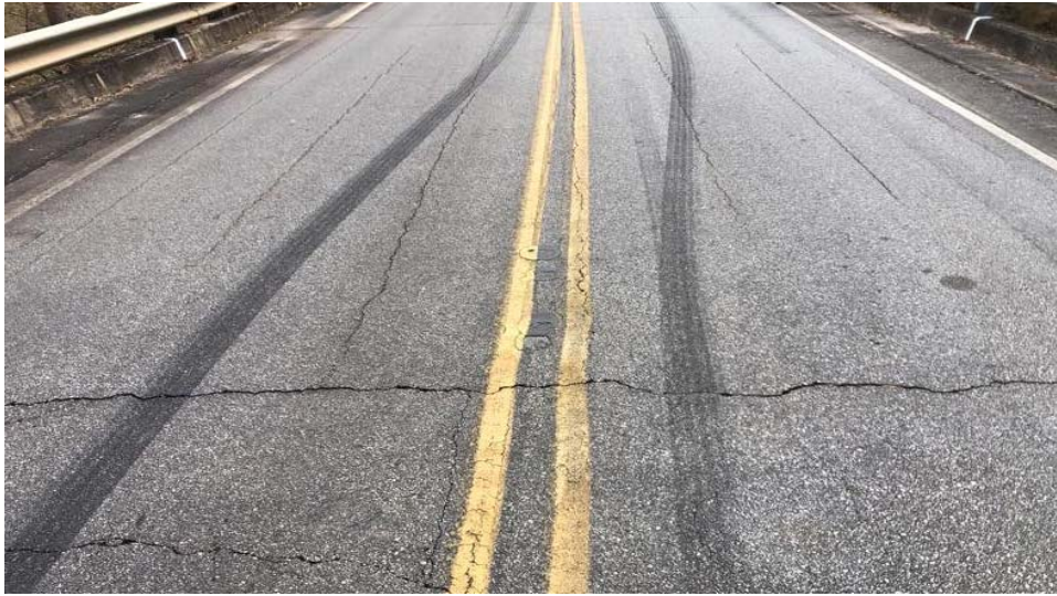
Reflective Cracking: Severe – DF = 0.5 Lane
