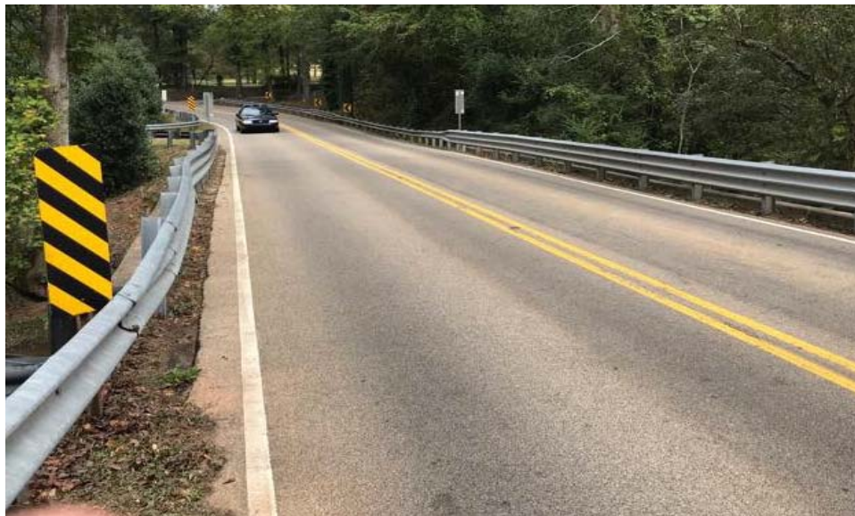
Figure 2 Bridge Deck Asphalt Overlay; None/Minor Reflective Cracking
