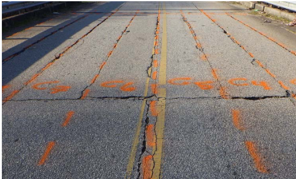
Figure 4 Bridge Deck Asphalt Overlay; Severe Reflective Cracking
