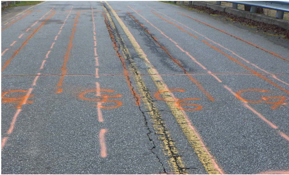
Reflective Cracking: Localized Severe - DF = 0.5 Lane
