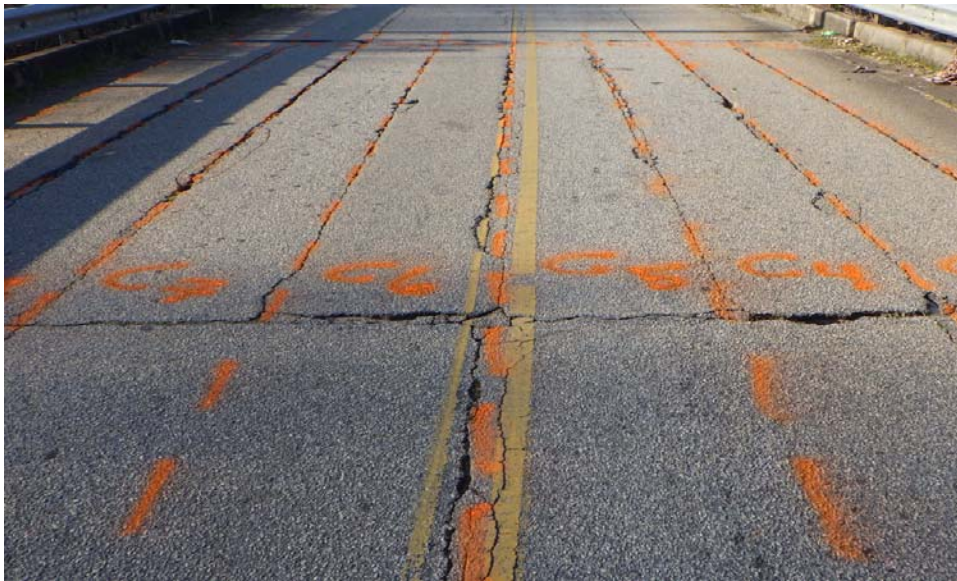
Reflective Cracking: Severe – DF = 0.5 Lane
