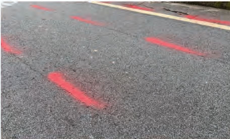
Reflective Cracking: Moderate - DF = 0.35 Lane
