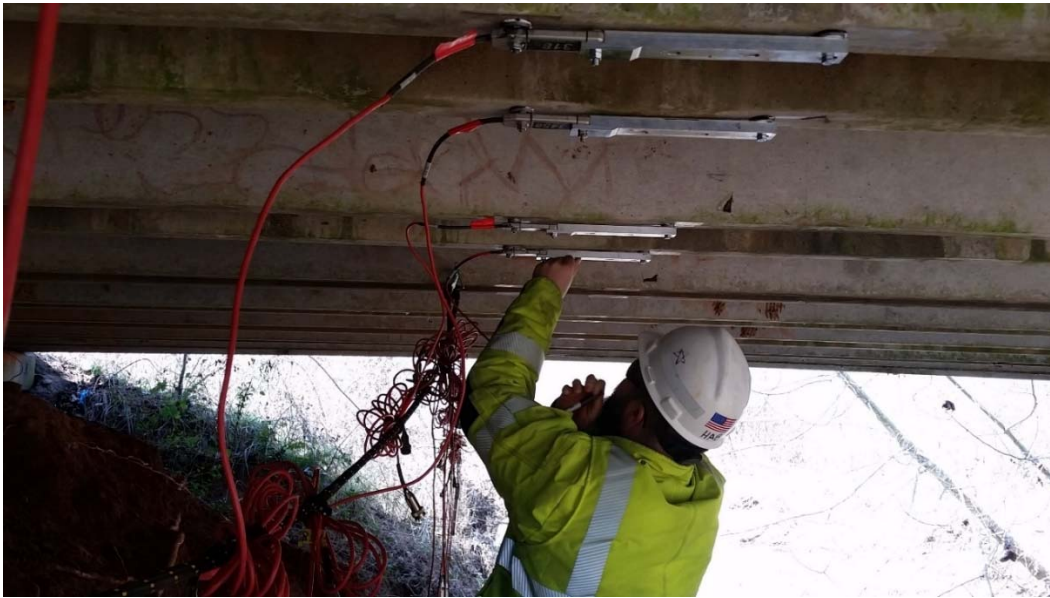
Figure 12: Strain Gauge Installation
