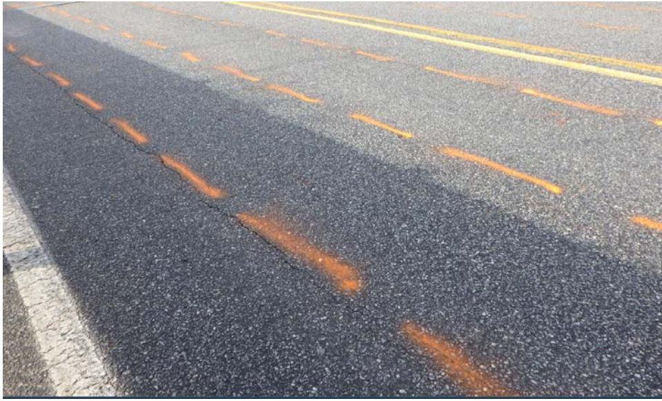
Reflective Cracking: Moderate - DF = 0.35 Lane
