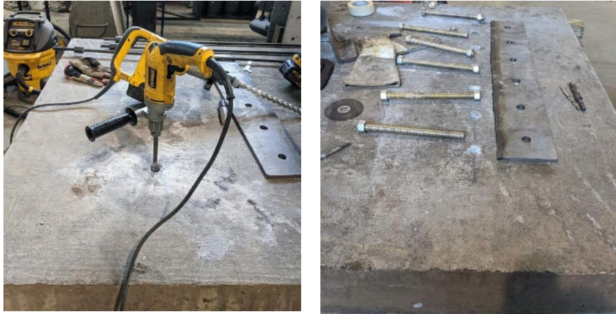
Figure 3.14 Hammer Drilling (left) and threaded rods and steel plate ready to be placed on the slab (right).
