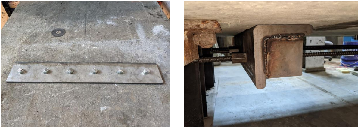
Figure 3.15 Installation of steel plates (left) and installation of steel angles and DYWIDAG threadbars (right).
