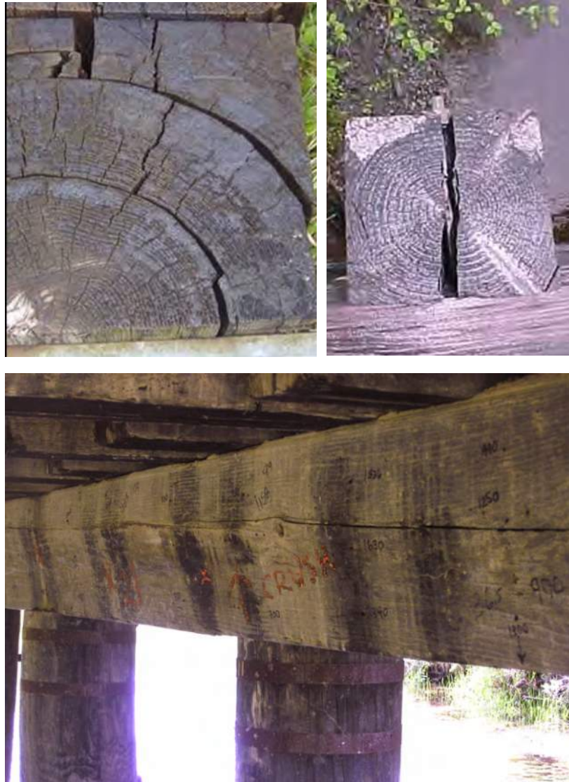
Figure 3.7 Timber members showing various types of deterioration. Top left shows ring shake. Top right shows severe through splits. Bottom picture is of a long horizontal split provides an opportunity for moisture passing through the timber deck to enter the cap, leading to substantial decay.
