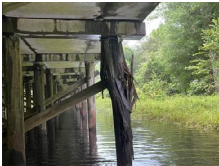
Figure 3.1 Failed timber pile due to internal decay of the pile at a cross-frame through bolt.
