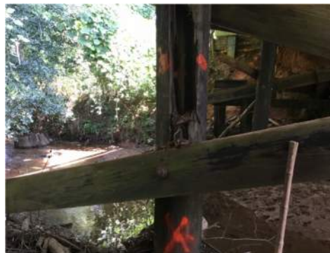
Figure 7.2 Exterior Pile with > 50% Decay, Drilling Not Needed (Critical Finding/A Flag per Figure O.3 in App O)
