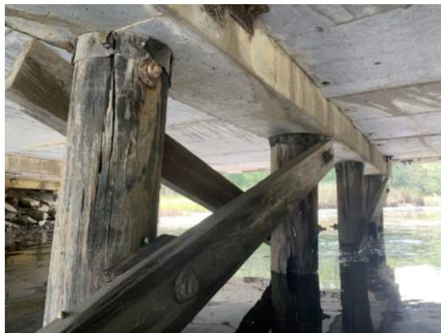
Figure 1.0 Example of a Timber Pile Bridge (Timber Piles under Reinforced Concrete Cap)
