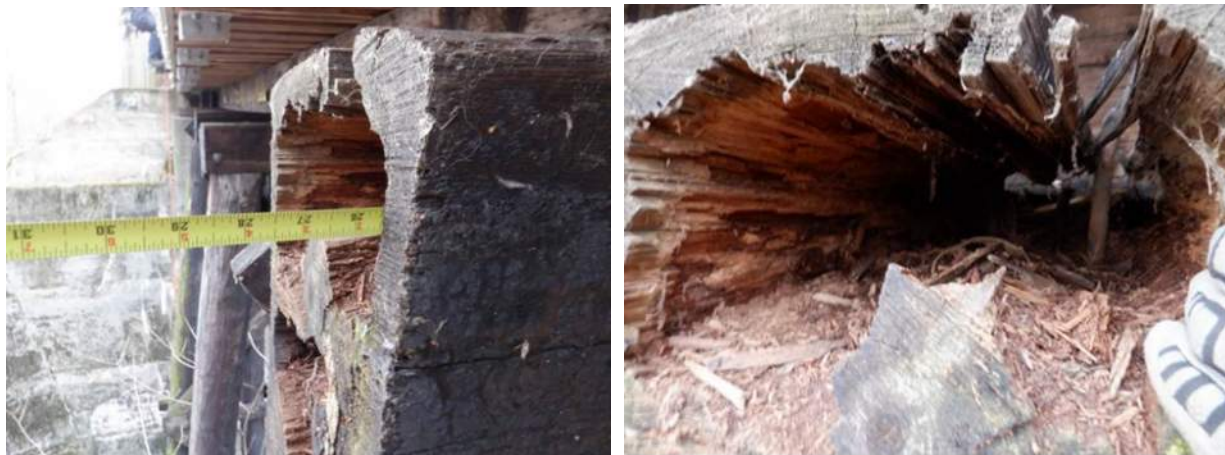
Figure 3.3 Localized collapse of a timber bent cap.
