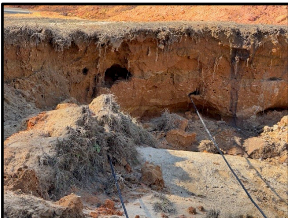
Pointing Northwest B-1 Bank from Central Culvert Tube, Exposed Cables
