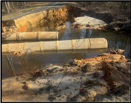
Pointing Southeast From B-1 Bank (Exposed Communication Cables)
