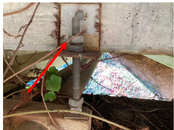
Photo 6 LBP on Utility Bracket attached to the Underside of the Bridge on the South Side.
