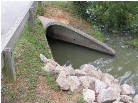
Use Pipe Flared End Section when specified in the plans or special provisions.
