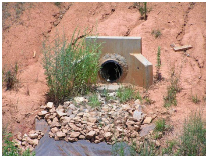
Use Pipe Wingwall Section when specified in the plans or special provisions.
