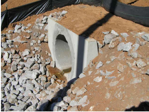
Use Pipe Straight Headwall (719-605-00) when specified in the plans or special provisions. Use straight headwall only in locations where pipe exposed end does not face the direction of traffic.
