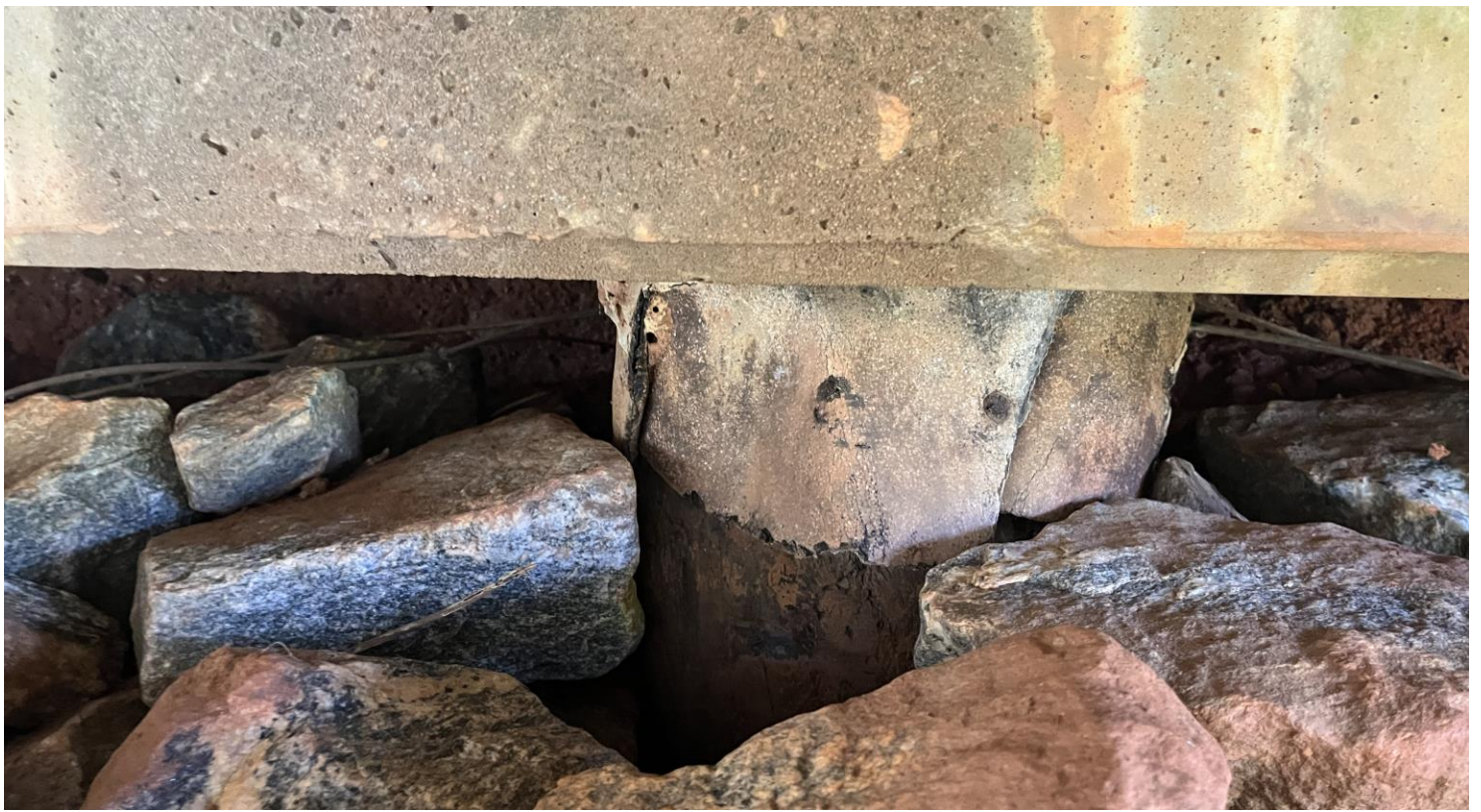
PHOTO # 5 View of HA #1 Thick shingle vibration dampener.
