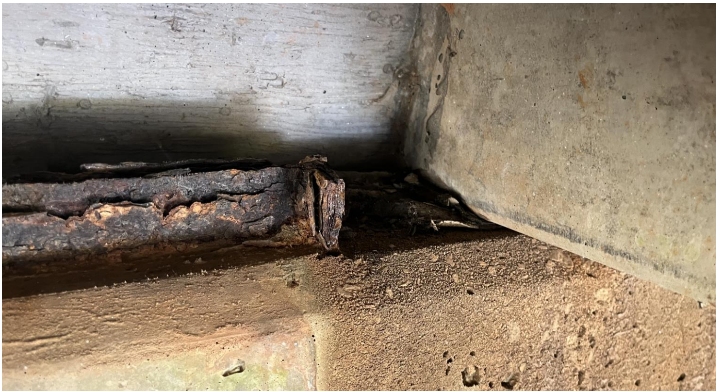
PHOTO # 6 View of HA #2 Thin felt vibration dampener.
