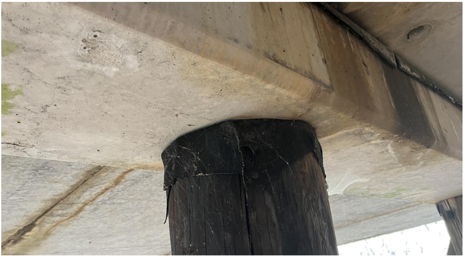
PHOTO # 5 View of HA #2 Thin felt vibration dampener.
