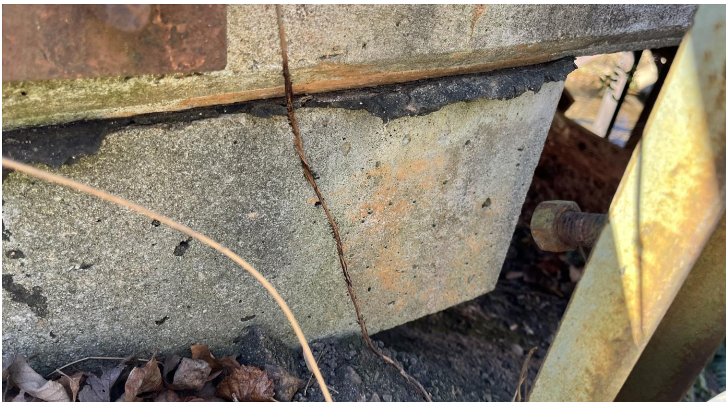
PHOTO # 3 View of HA #1 tar vibration dampener
