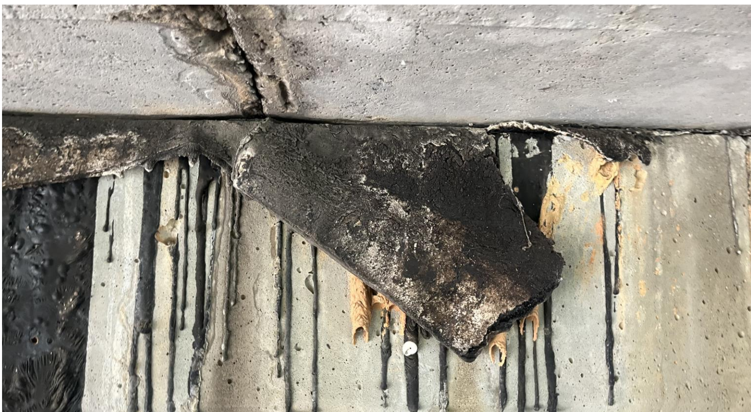
PHOTO # 4 View of HA #2 Thick tar and shingle vibration dampener.
