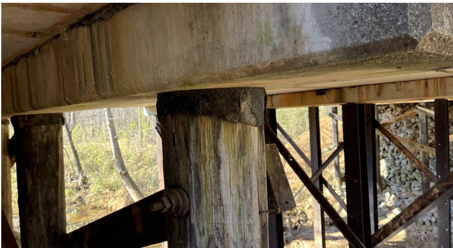
PHOTO # 4 View of HA #2 thin felt vibration dampener.
