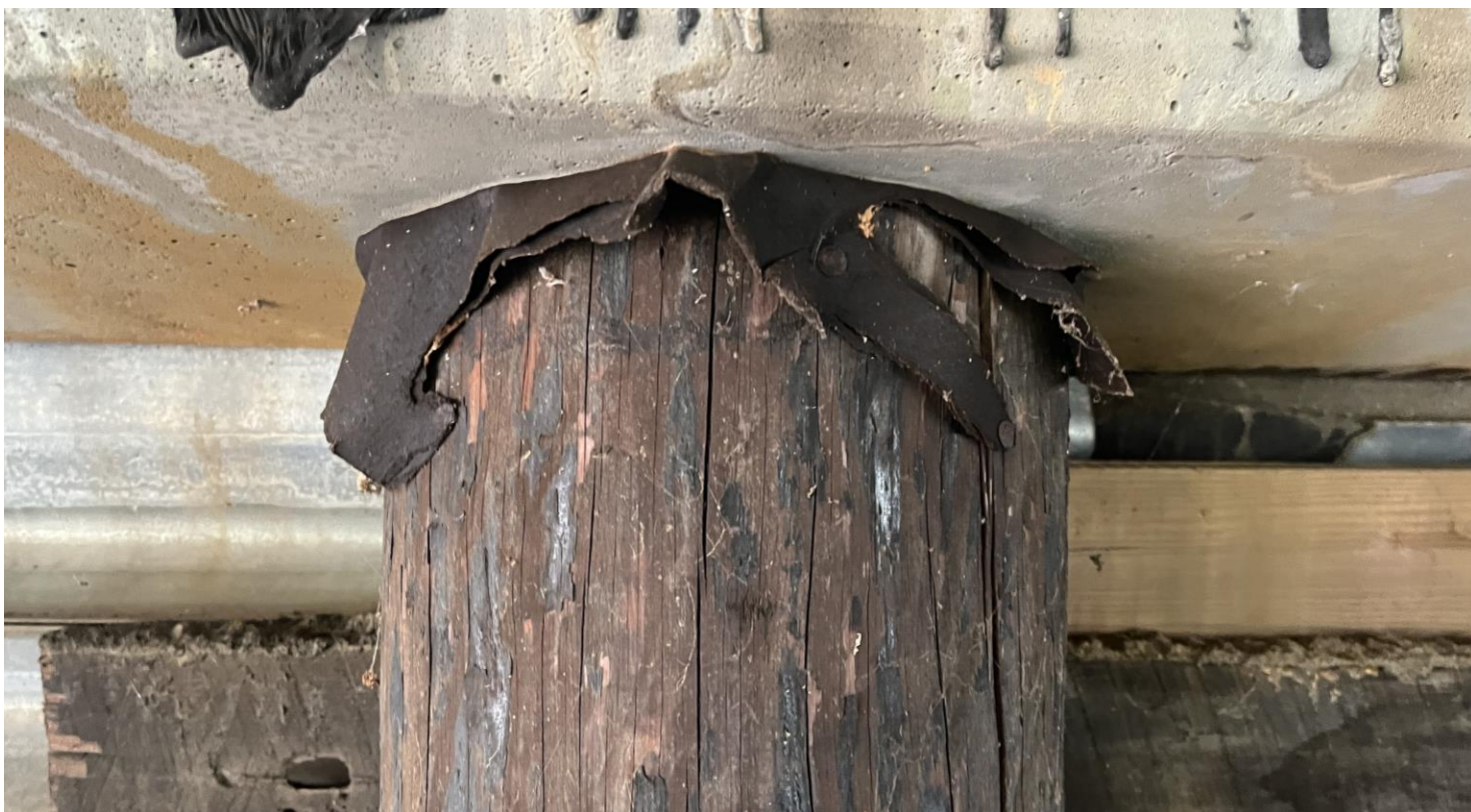
PHOTO # 3 View of HA #1 Thin felt vibration dampener between the piers and pier caps.
