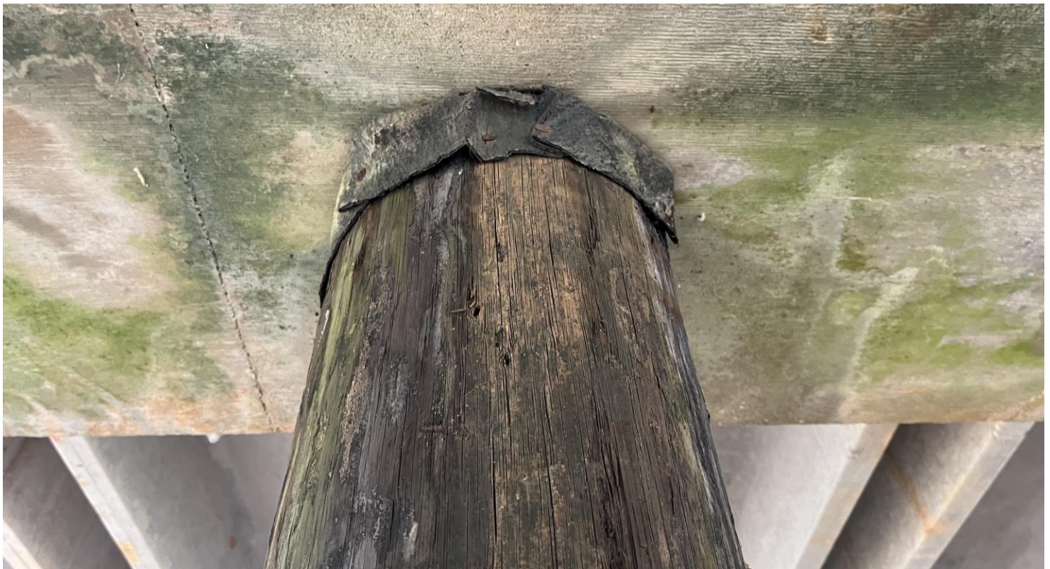
PHOTO # 4 View of HA #1 thick shingle vibration dampener.
