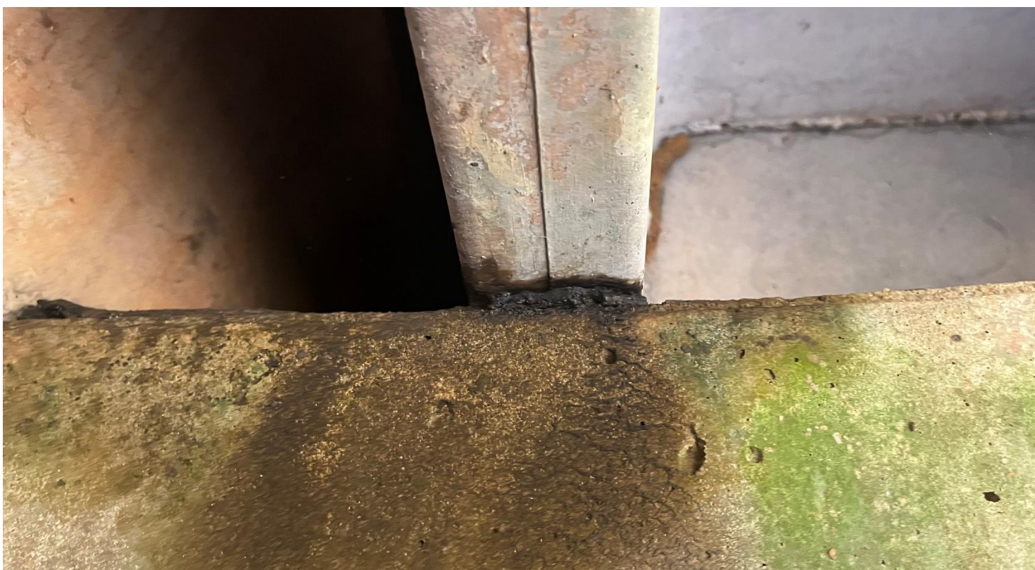
PHOTO # 6 View of HA #2 Tar and shingle vibration dampener rolled.
