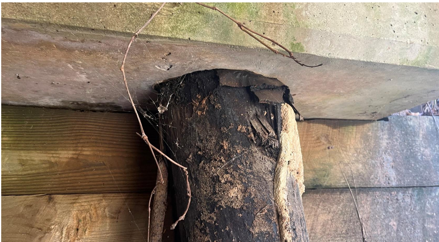
PHOTO # 5 View of HA #1 Tar and shingle vibration dampener poured.
