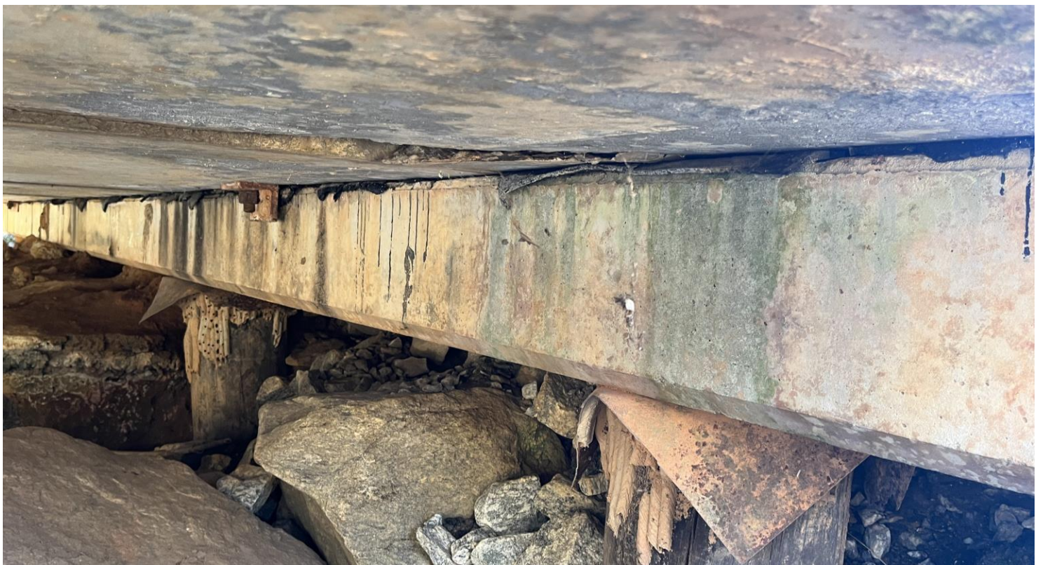
PHOTO # 4 View of HA #1 Thick tar and shingle vibration dampener.
