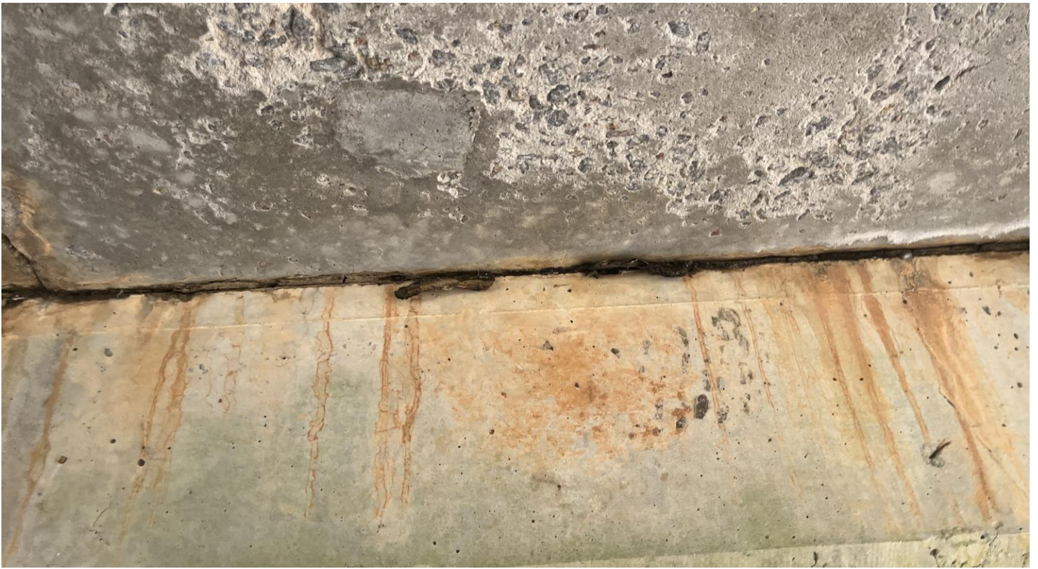
PHOTO # 5 View of HA #1 Thick tar and felt vibration dampener.
