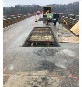
Photo 1: Typical bridge deck repair
