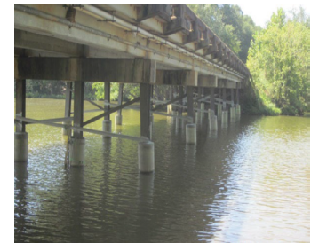
Photo 2: Pile jackets added to steel pile under the bridge
