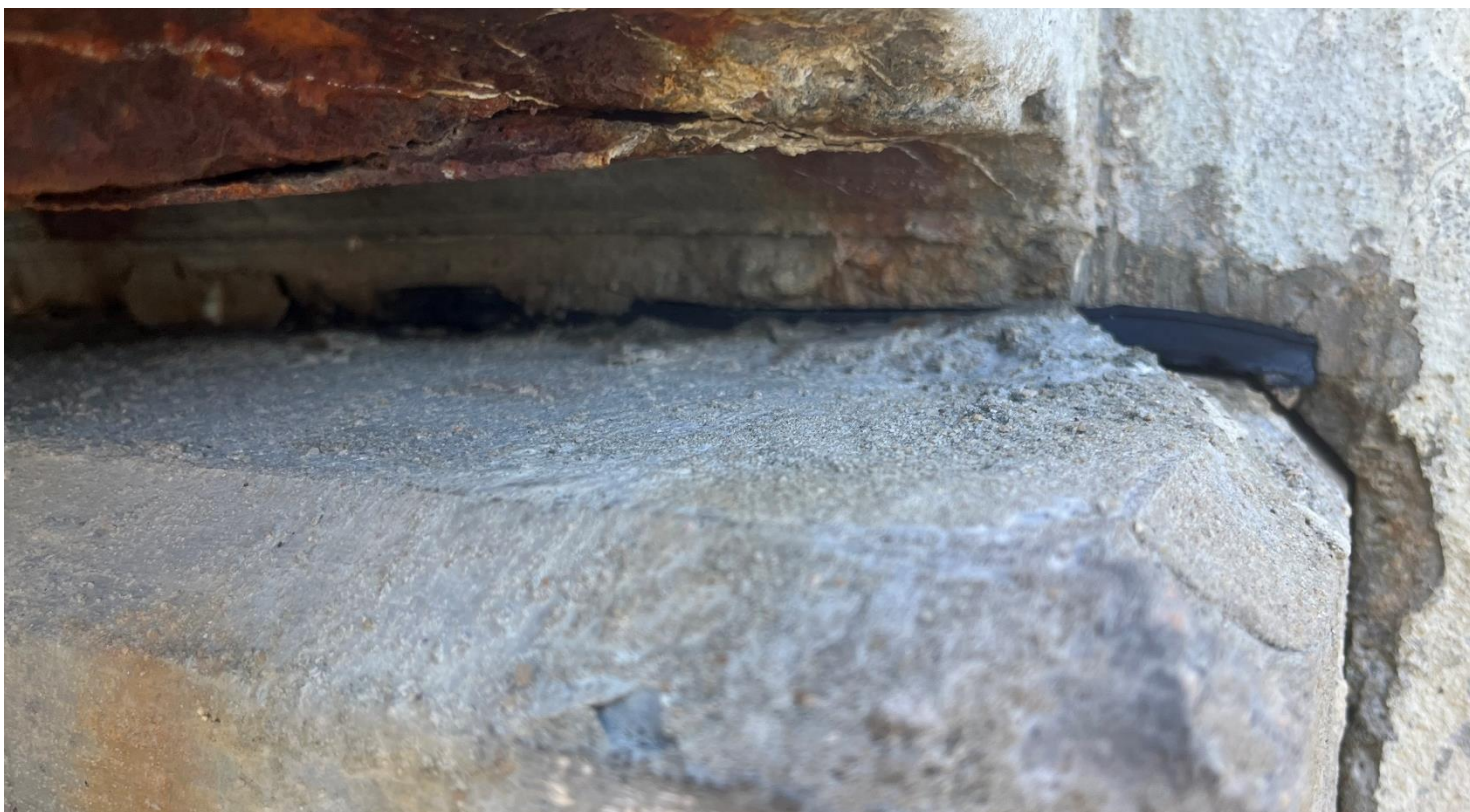
PHOTO # 5 View of rubber vibration dampener between pier cap and decking, not suspect.
