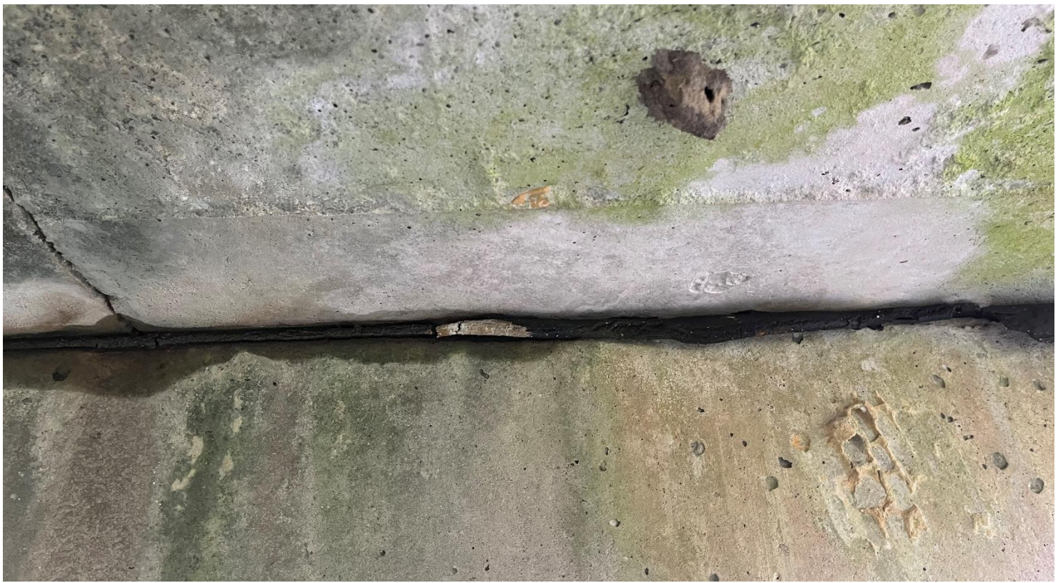
PHOTO # 5 View of HA #2 Thick tar vibration dampener between pier cap and decking.
