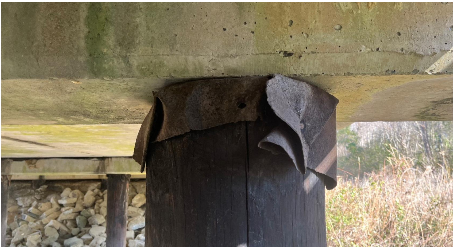
PHOTO # 4 View of HA #1 thin felt vibration dampener between pier and pier cap.
