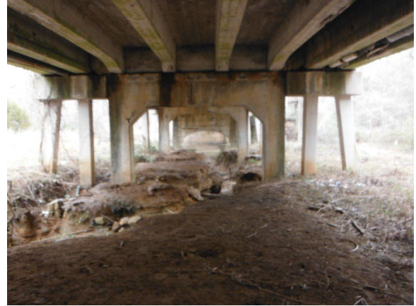
Photo 2. Underside View of Bridge with view of additions on each side of Bridge.
