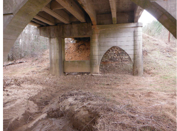
Photo 2. Original Bridge and Addition, Underside View.
