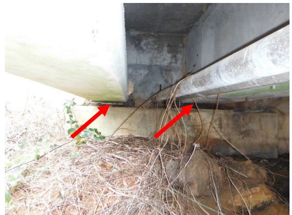
Photo 6. LBP on Bridge Beam Bearing Plates.
