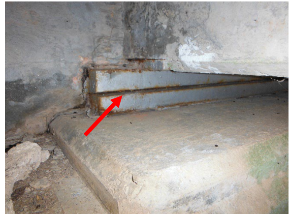
Photo 4. Steel Bearing Plates Positive for LBP.
