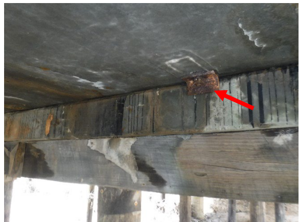
Photo 6. Positive LBP on bridges deck to bent cap anchor bracket.
