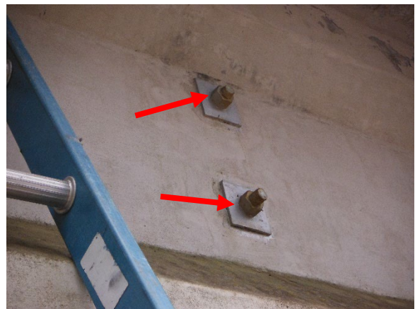
Photo 6. Bridge Tie-Rod Washers Positive for LBP.
