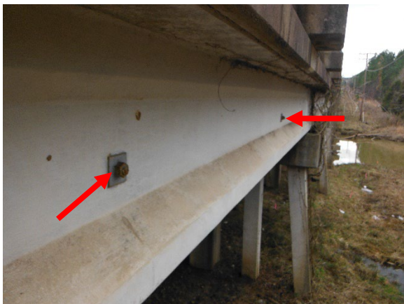
Photo 5. LBP on Bridge Tie-Rod Washers.
