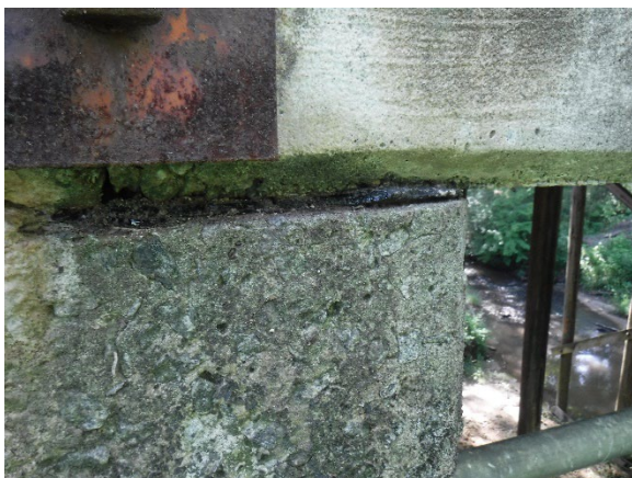
Photo 5. Bearing Pad Material.
