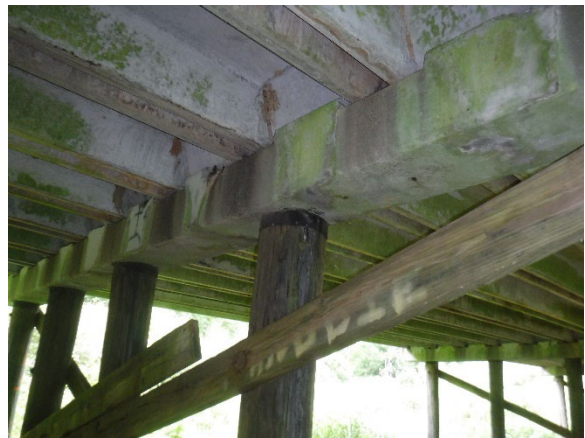
Photo 4. Timber Pile Cap Felt.
