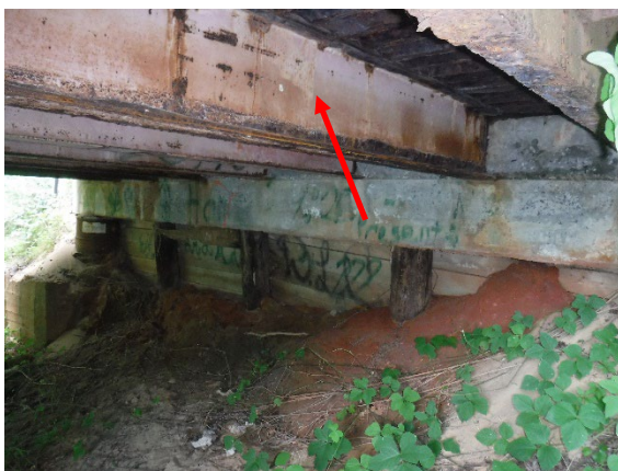
Photo 5. LBP on Orange Beams.
