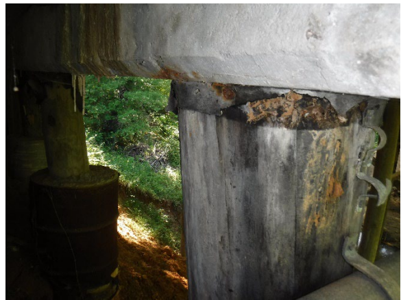
Photo 4. Timber Pile Cap Felt.
