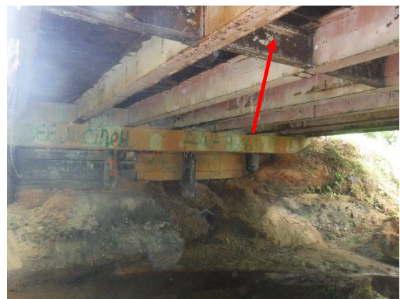
Photo 6 LBP on Orange Cross Braces.
