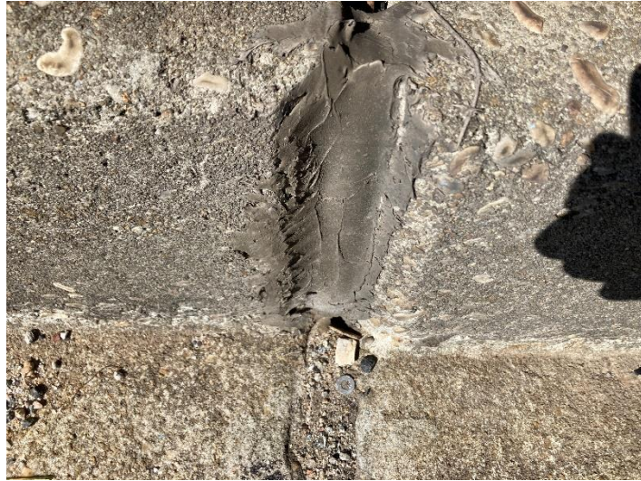
Photo 5: HA #2E and #2W Putty expansion joint (05780 + 05785)
