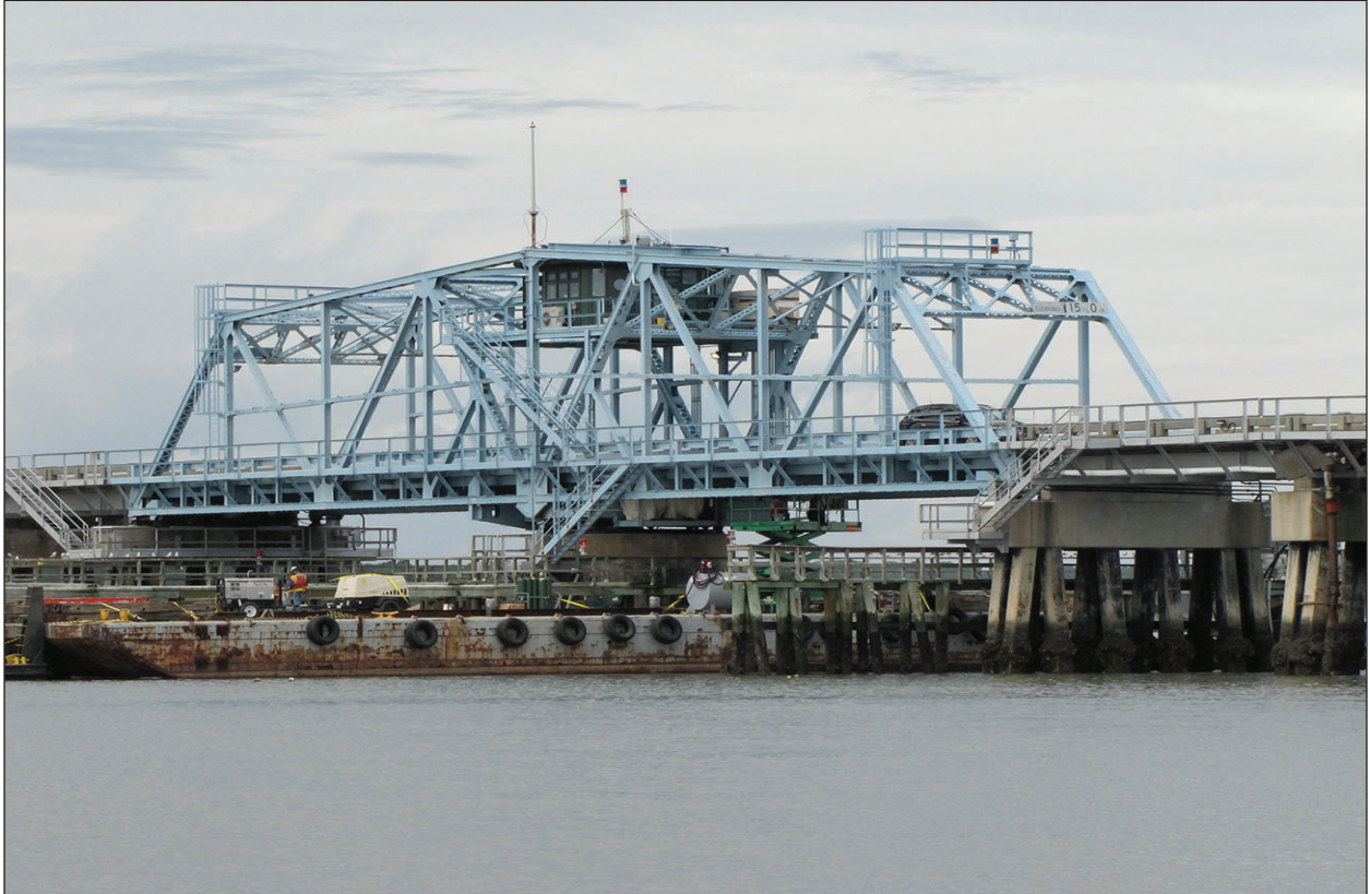
Figure 4.2 Resource 5070 Harbor River Bridge central pivoting section, facing northwest.
