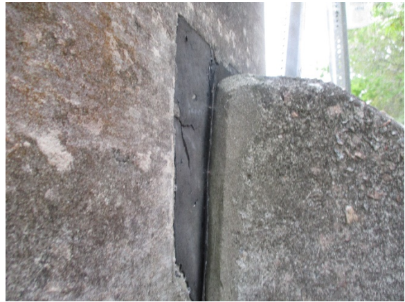
Photo 4. Expansion Joint Material.
