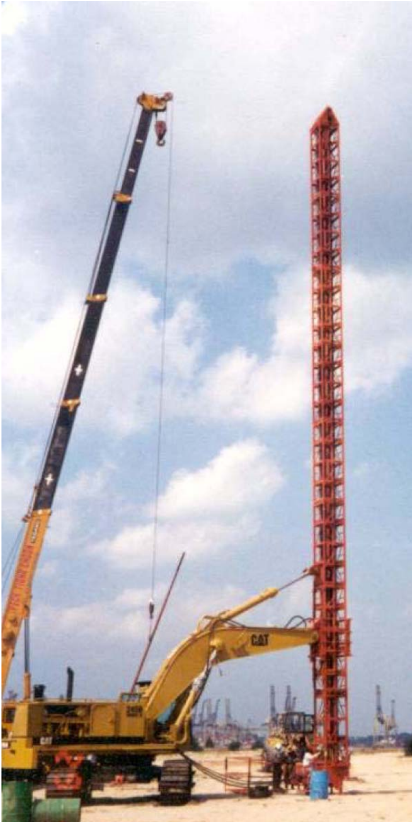
Photograph of Excavator-Mounted Wick Drain Rig.
