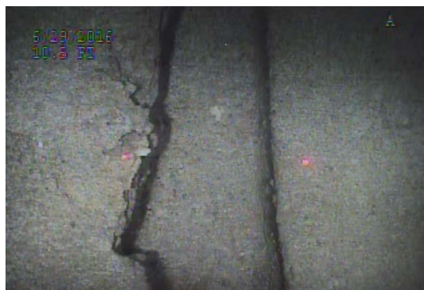
11' - Joint Offset/Crack > 12"
