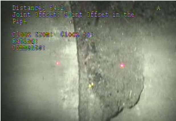
64.2' - JOINT OFFSET/BROKEN
