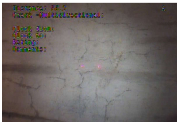
55' - Multidirectional Crack
