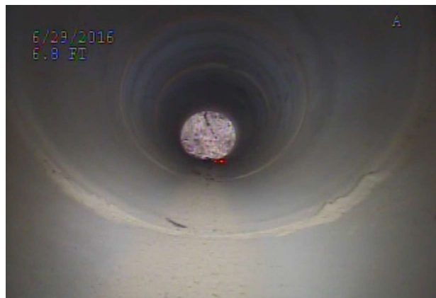
Pipe is in good condition
