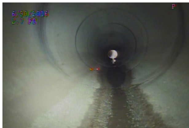
Pipe is in good condition
