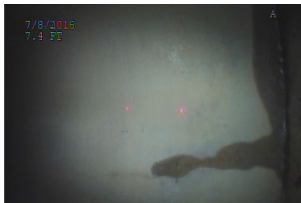
7' - Multidirectional Crack
