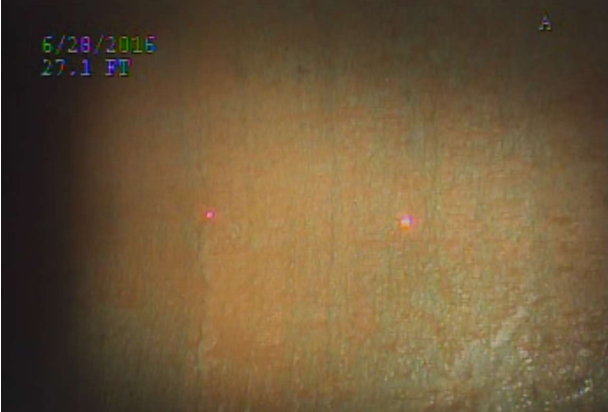
27.1' - CIRCUMFERENTIAL CRACK
