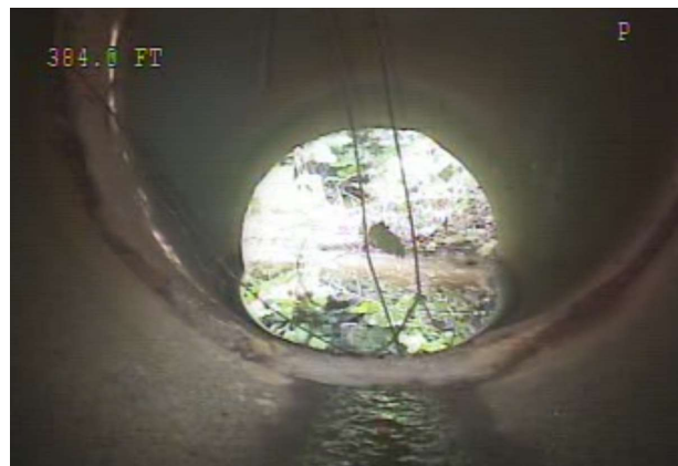
388.4' - Pipe collapsed
