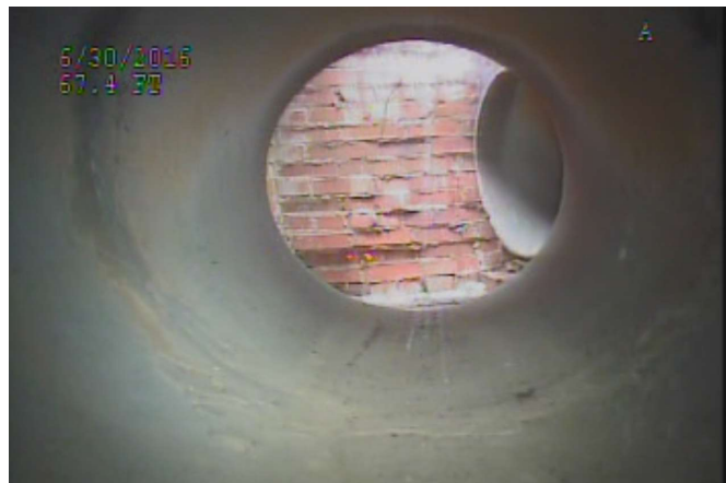
Pipe is in good condition
