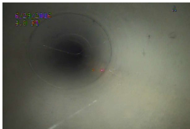
Pipe is in good condition
