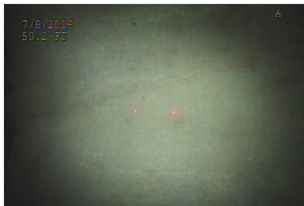
50' - Multidirectional Crack
