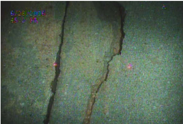
45.2' - Circumferential Crack
