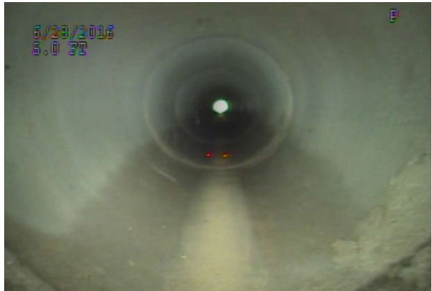
Pipe is in good condition
