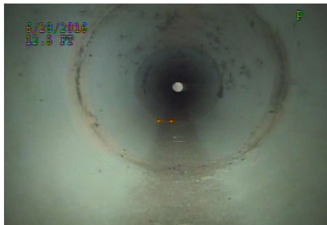
Pipe is in good condition
