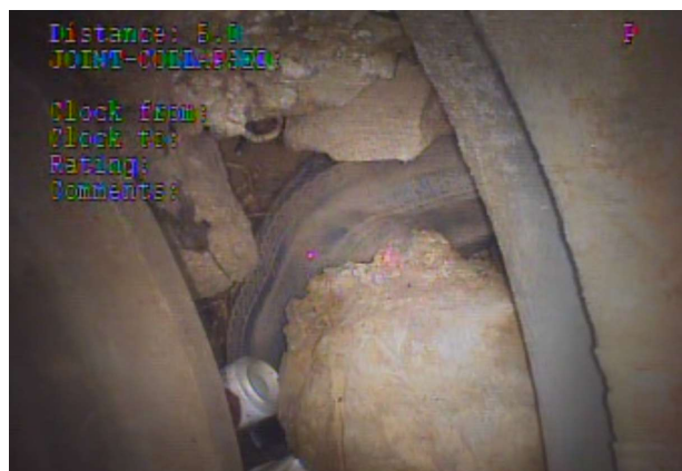
5' - Joint Collapsed
