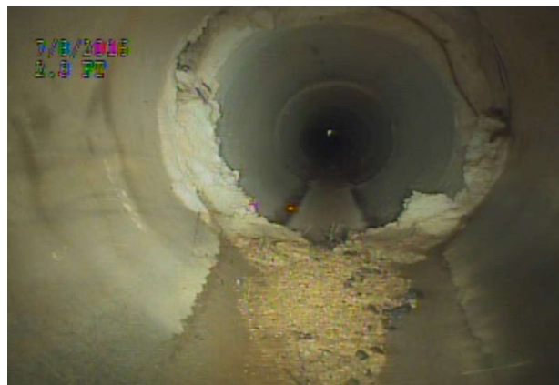
5' - Joint Collapsed
