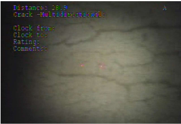
28.9' - Multidirectional Crack
