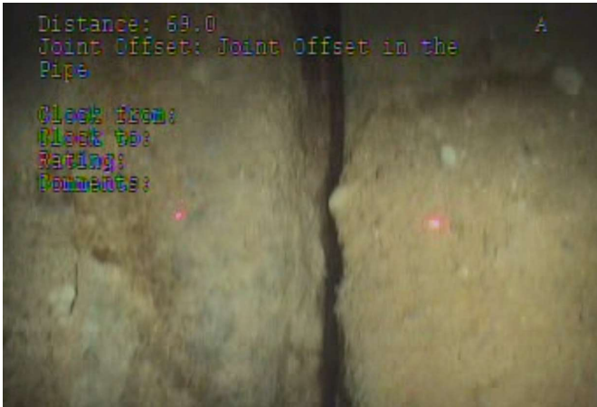
69' - JOINT OFFSET IN PIPE
