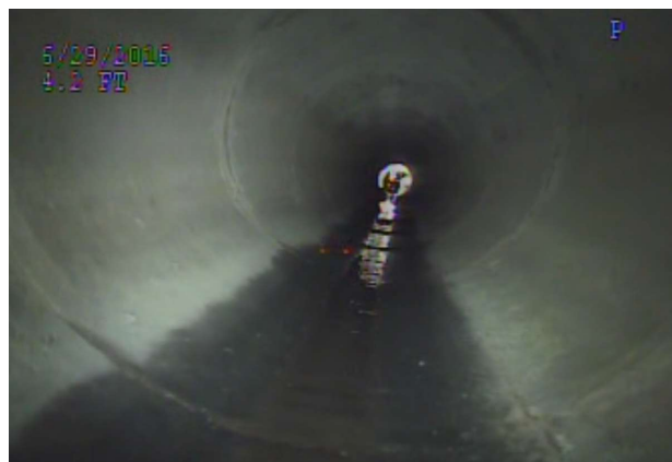
Pipe is in good condition
