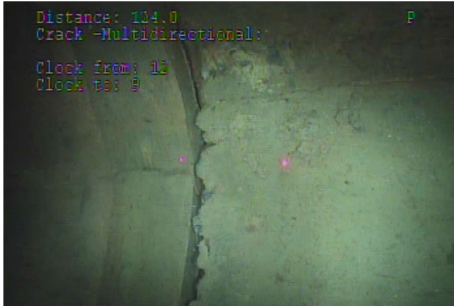
124' - MULTIDIRECTIONAL CRACK
