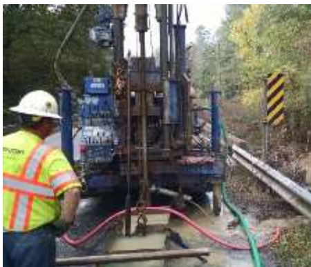
Photo 1. Drill rig at STB-1 (SC-34)
