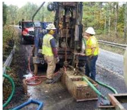
Photo 2. Drill rig at STB-2 (SC-34)
