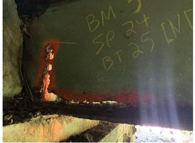
Typical section loss with holes on web. See table condition for more details
