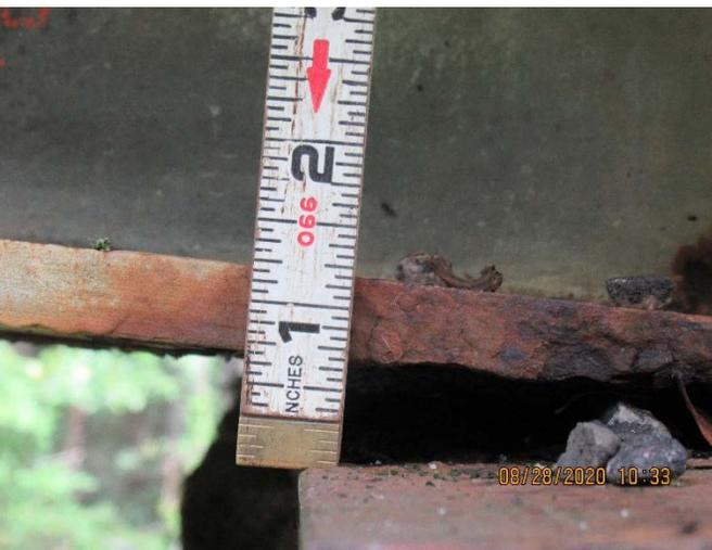
PHOTO #10 BM6 OF SP22 AT BT23= BEARING GAP
