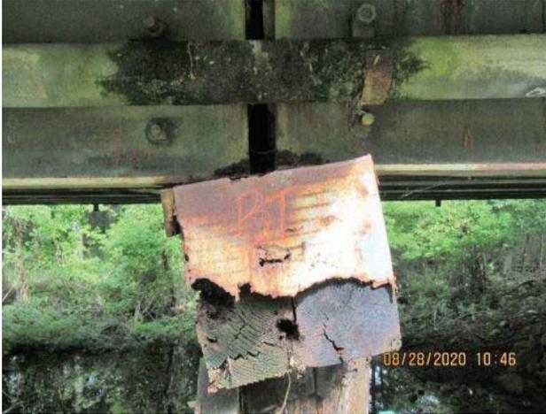
Rotation on bent 23 cap under beams 5 and 6
