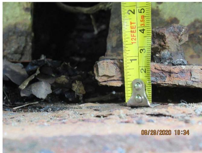
PHOTO #11 BM6 OF SP23 AT BT23= BEARING GAP
