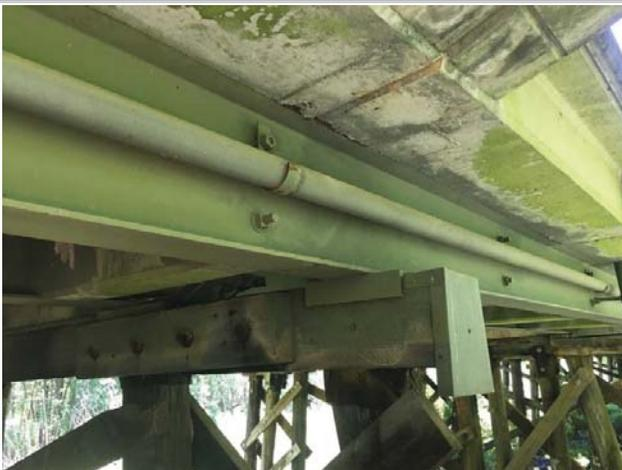
Girders continuous over every other bent. 12 (2) span continuous.
