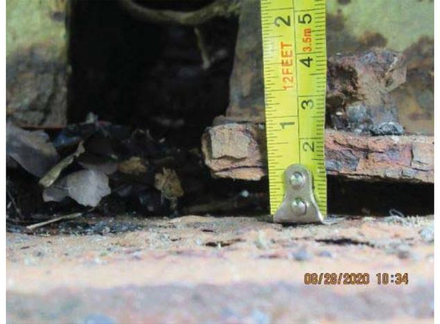
Gap between beams and cap at bent 23
