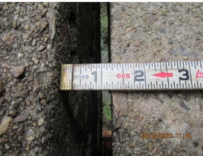
PHOTO #3 CURB GAP OVER BM AT BT23=
