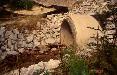
For all exposed crossline pipe ends, when an end treatment is not specified in the plans, use **Pipe Riprap Protection** (804-3xx-xx). For flexible pipe larger than 24" diameter, install pipe straight headwall, pipe end structure, flared end section, or wingwall section in addition to riprap. For all exposed driveway pipe ends where no end treatment is specified in the plans, use **Pipe Riprap Protection** (804-3xx-xx) unless directed otherwise by the engineer.
